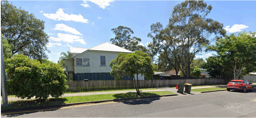
Figure 9: View of Site from Victor Street
