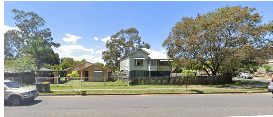
Figure 8: View of Site from Southern End of Persse Road
