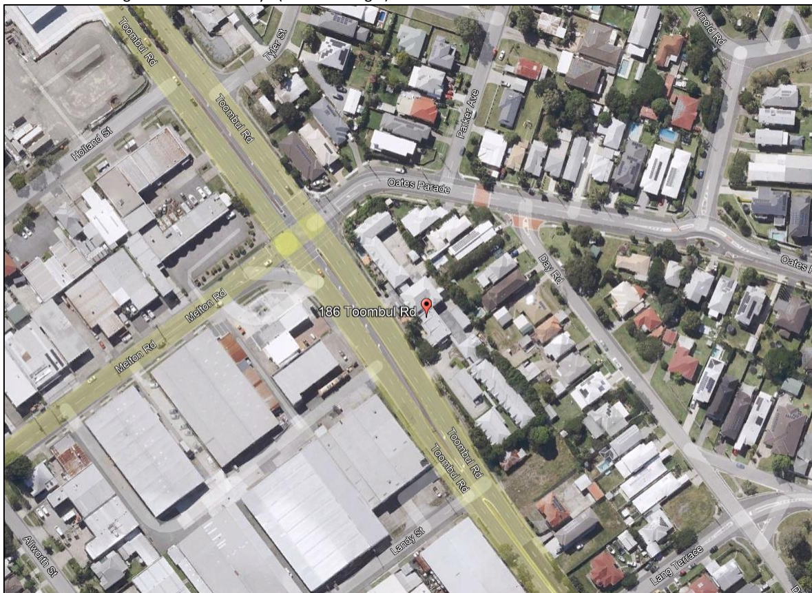
Plate 1.1: Showing the site and locality. (Source: Google).
