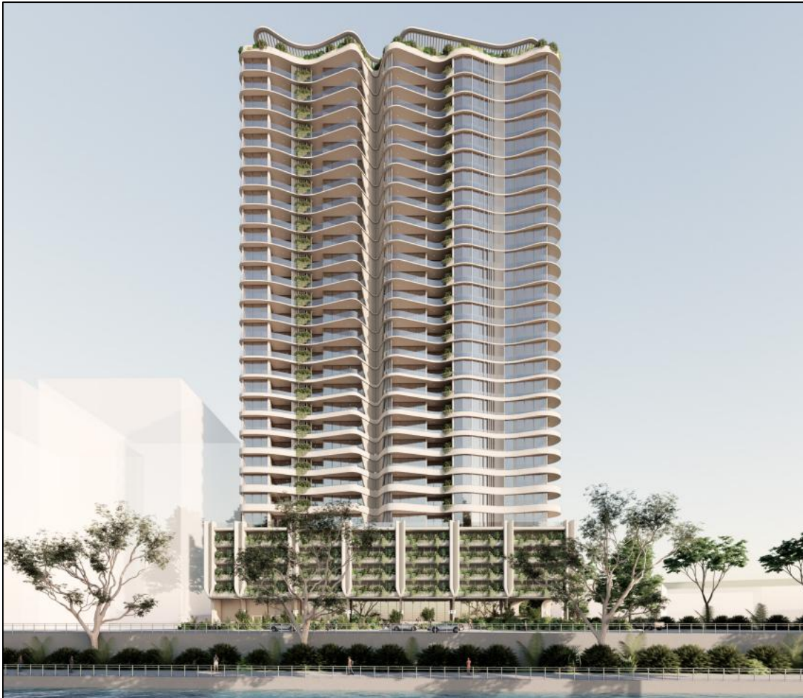
Figure 1: Rendered View of the changed proposal as viewed from the south-east (source: Plus Studio)
