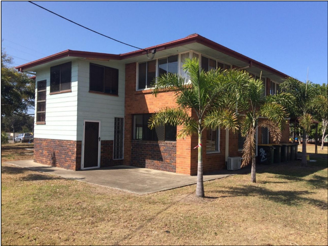
Photo 1: Existing house at 109 Lemke Rd, Taigum
