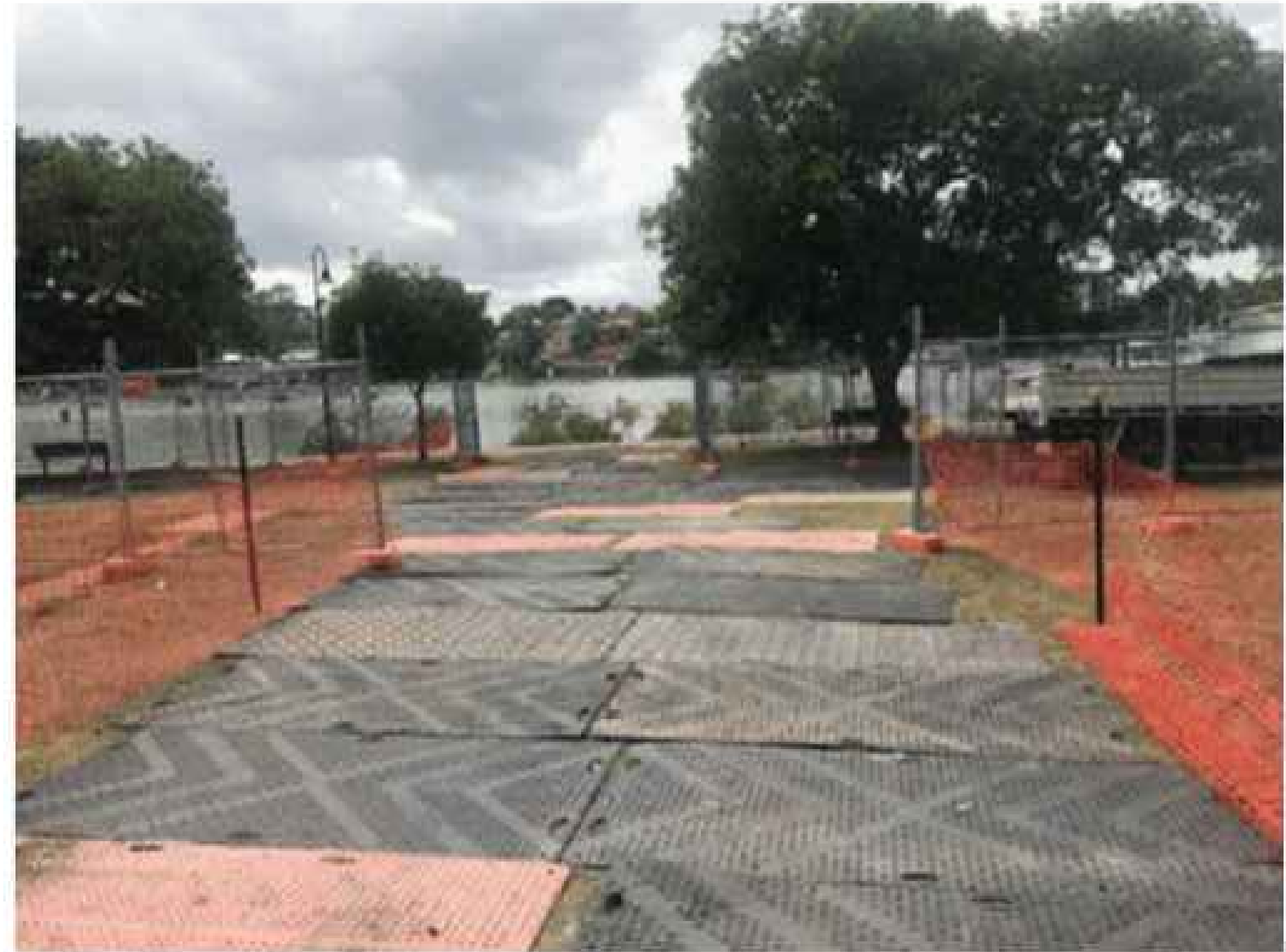
BRIDGING BOARDS OVER TREE PROTECTION ZONE (EXAMPLE)
