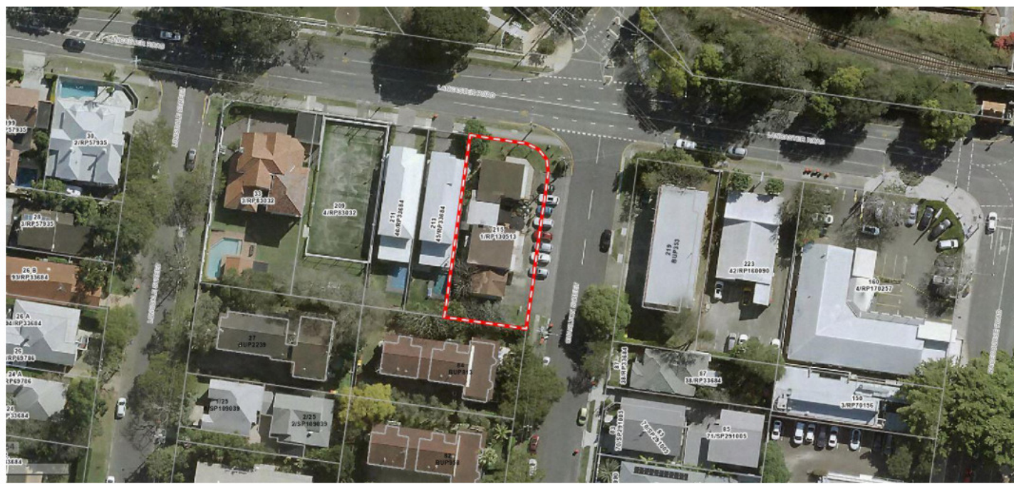
AERIAL VIEW - 2021 (SUPPLIED FROM BCC)
