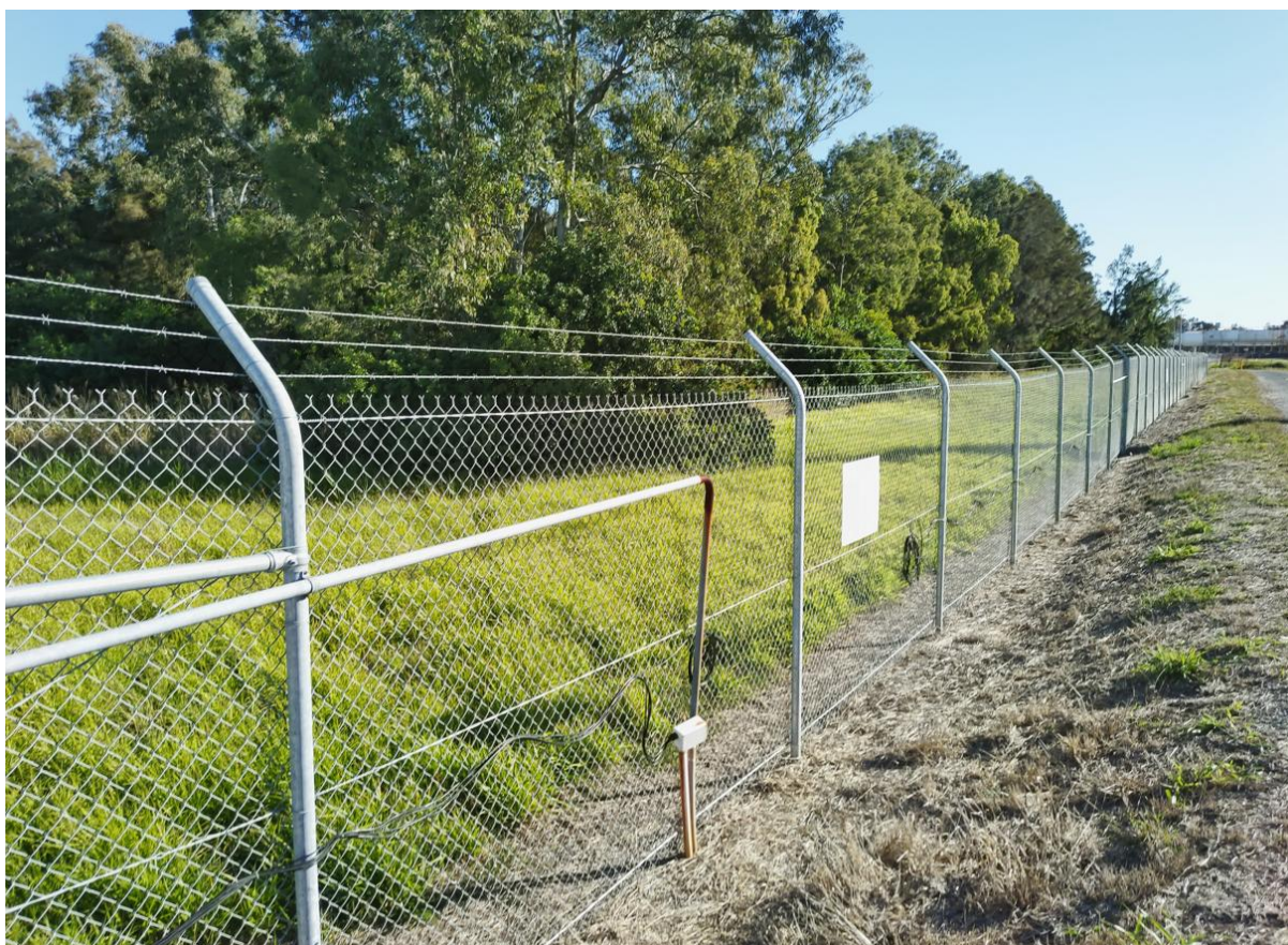
Photo 3: Bushfire hazard vegetation nearby
