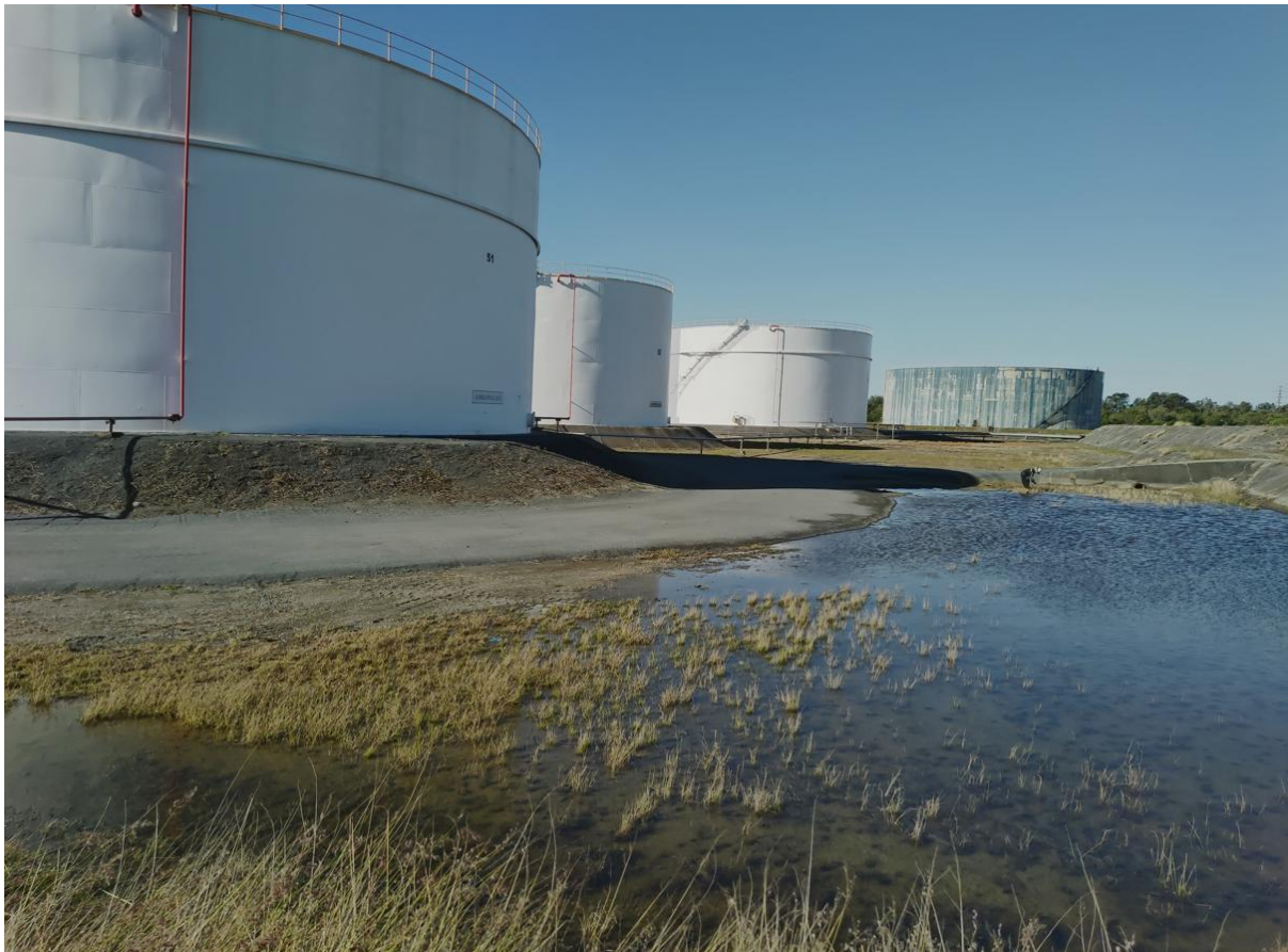
Photo 4: Low hazard areas
