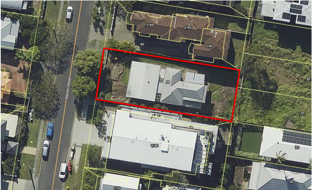
Figure 1: Aerial image of the application site (in red) and surrounding area. Source: Queensland Globe.
