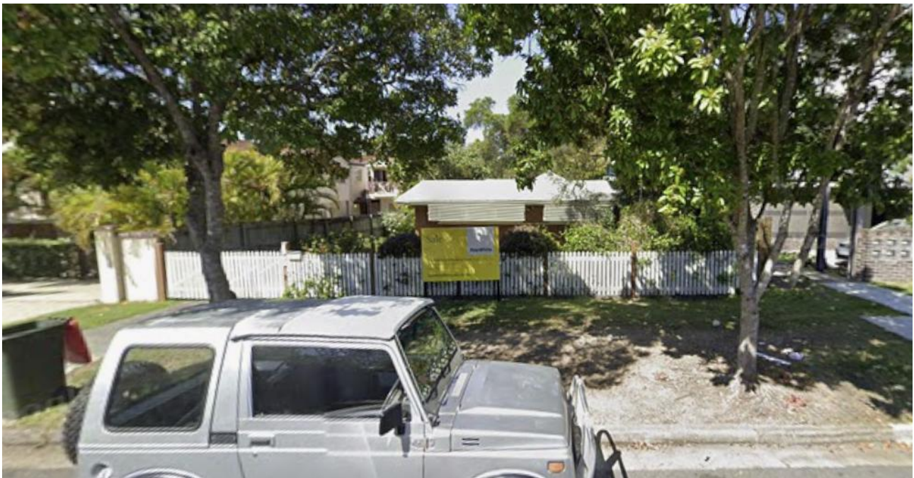
Figure 2: The existing dwelling (to be demolished) when viewed from Warren Street. Source: Google Streetview.
