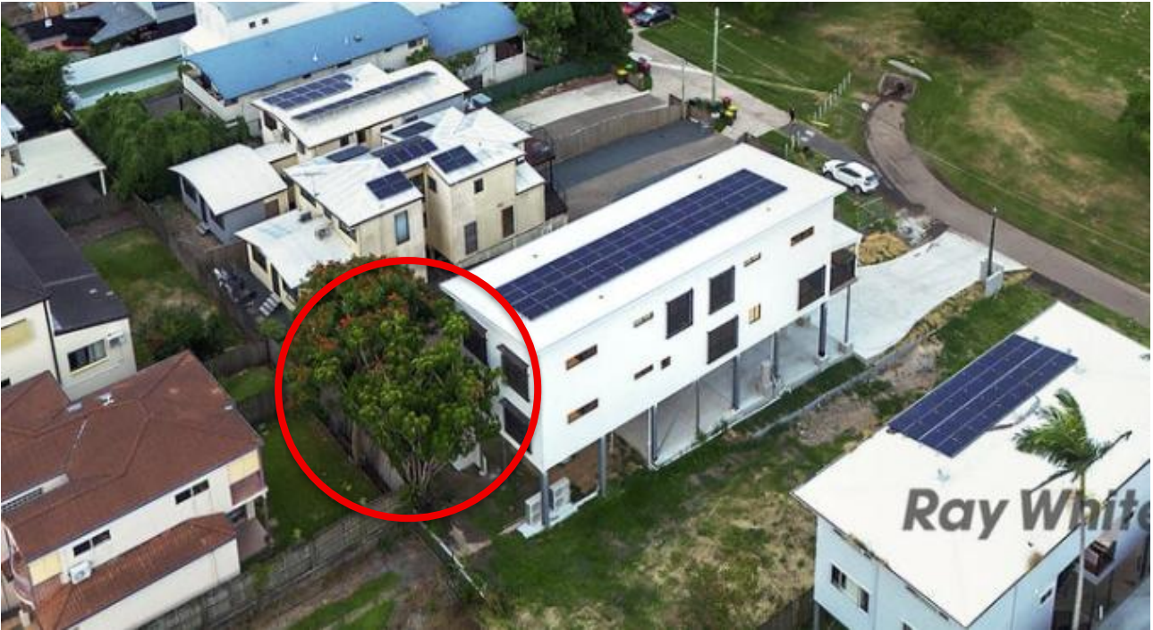
Figure 5: The existing tree at the rear of 89 Munro Street, which will provide sufficient screening between the buildings.
