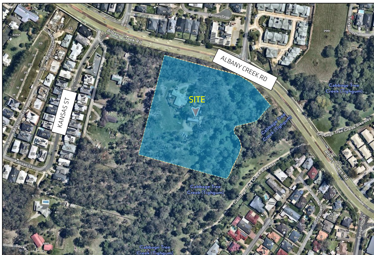
Figure 1 – Indicative Site Location (Nearmap, 2026)
