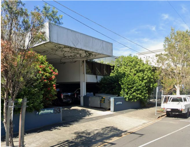
Picture 1 – North east
