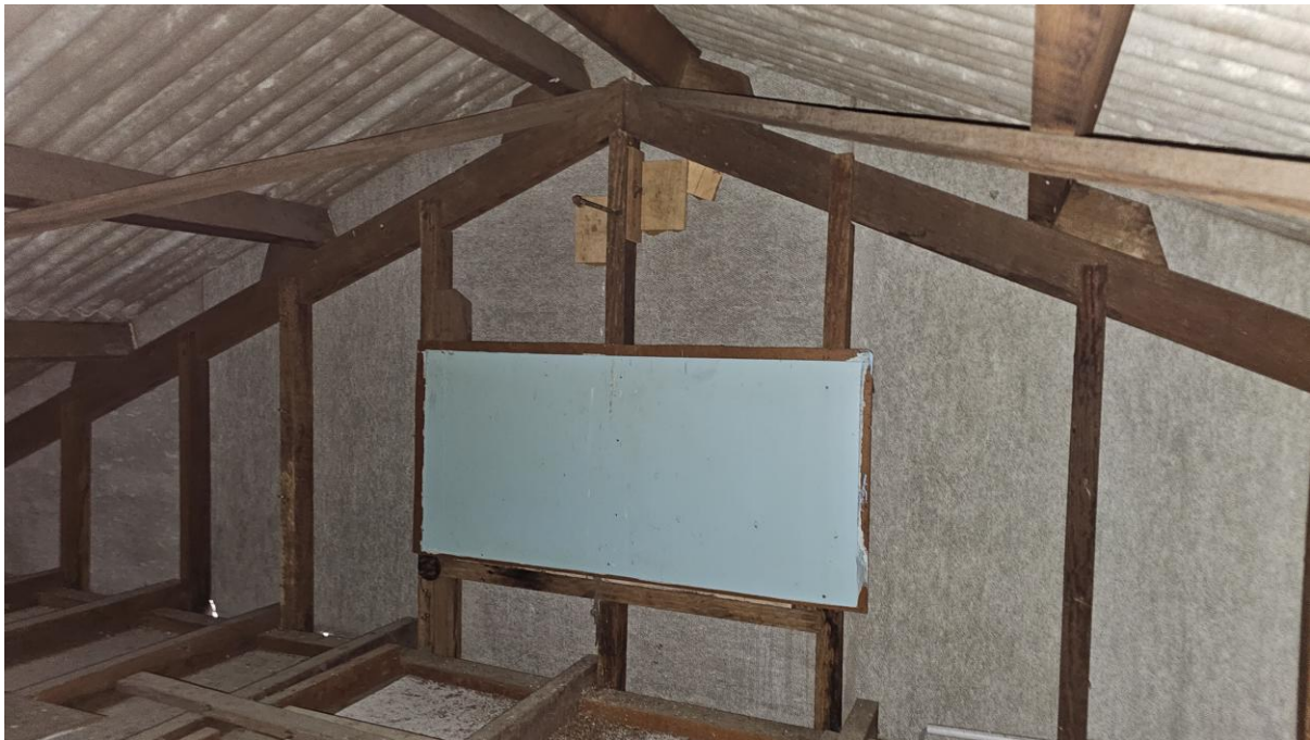
Photo 4: Gable End Wall
