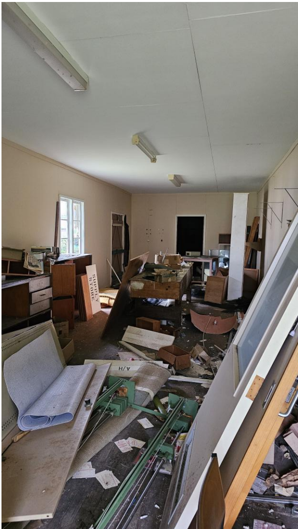
Photo 1 (Left): Internal of Building
