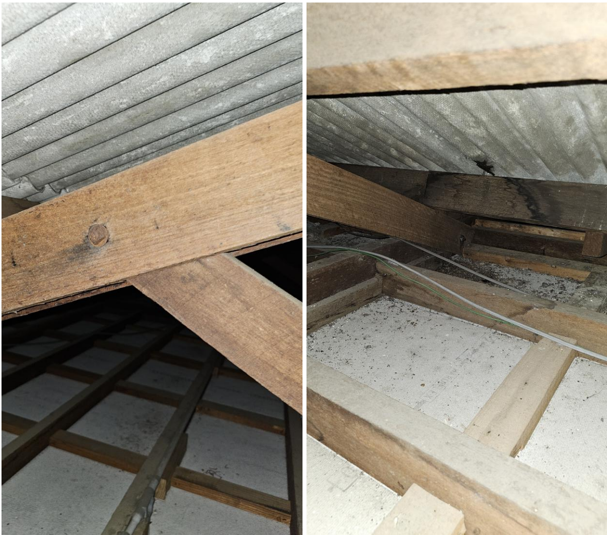
Photo 5 (Left): Bolt Connection Between Truss Members
