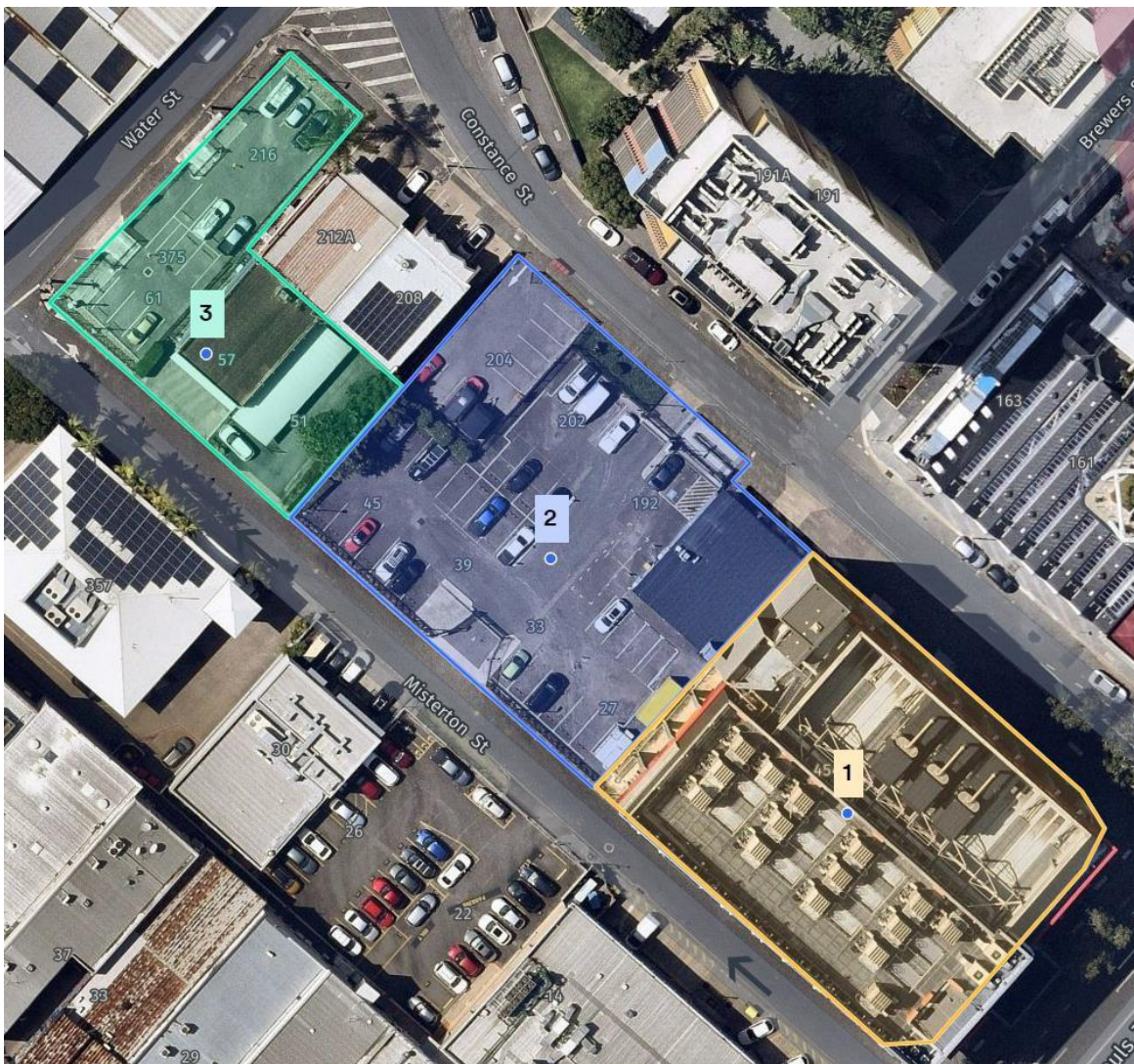
Figure 1: NEXTDC Innovation and Technology Precinct Stages Source: Nearmap, 2022
