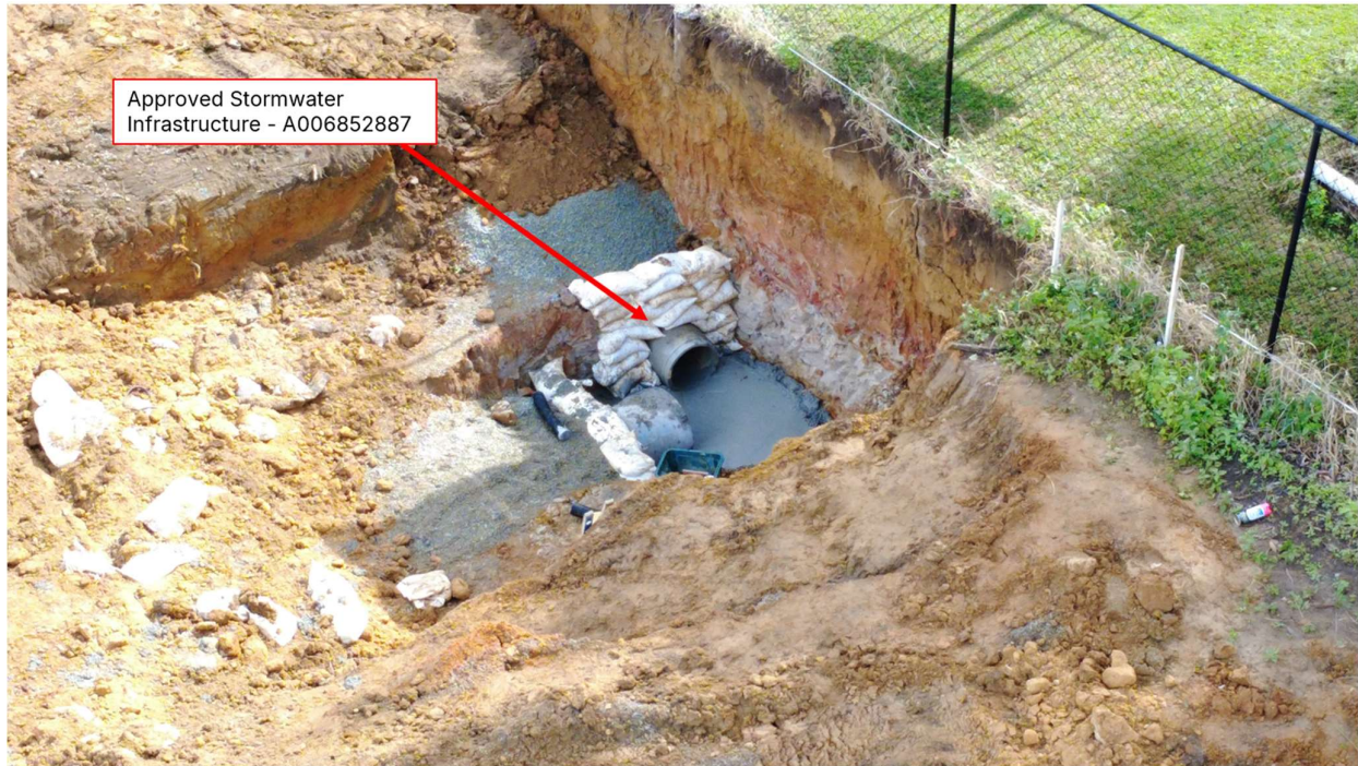
Figure 1 - Progress on downstream stormwater connection to south
