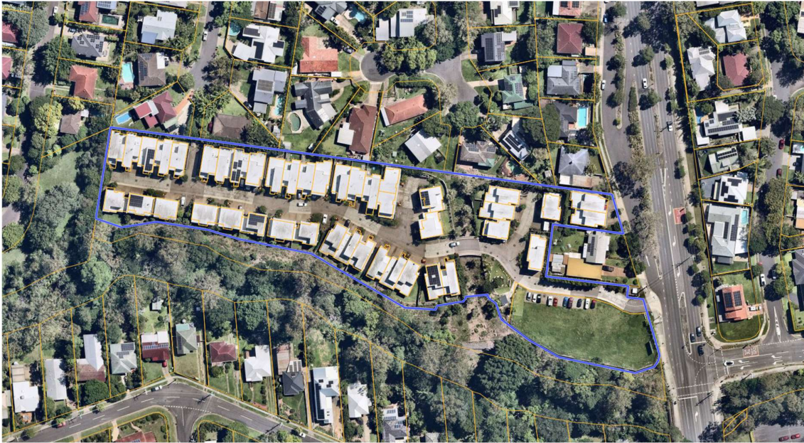
Figure 1 – Aerial Photo of Subject Site (dated June 2026) – demonstrating construction works onsite (Source: NearMap, 2026)
