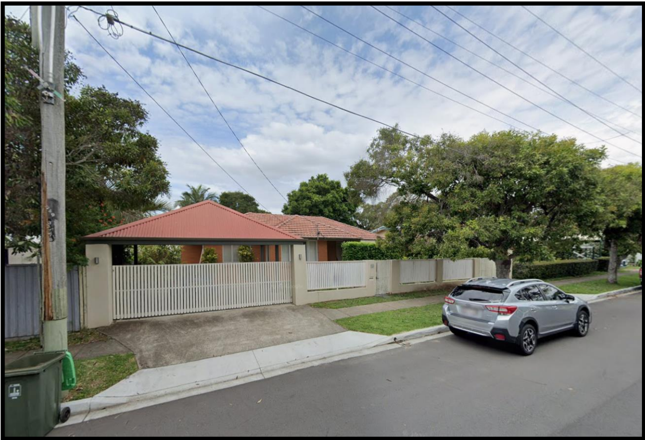
Figure 1 – 51 Wilmah St, Aspley frontage (Source: Google Streetview).
