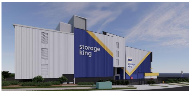
Picture 25 – Break in form, Buranda Street
