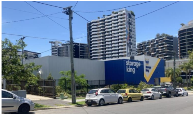
Picture 1 – Buranda Street Frontage
