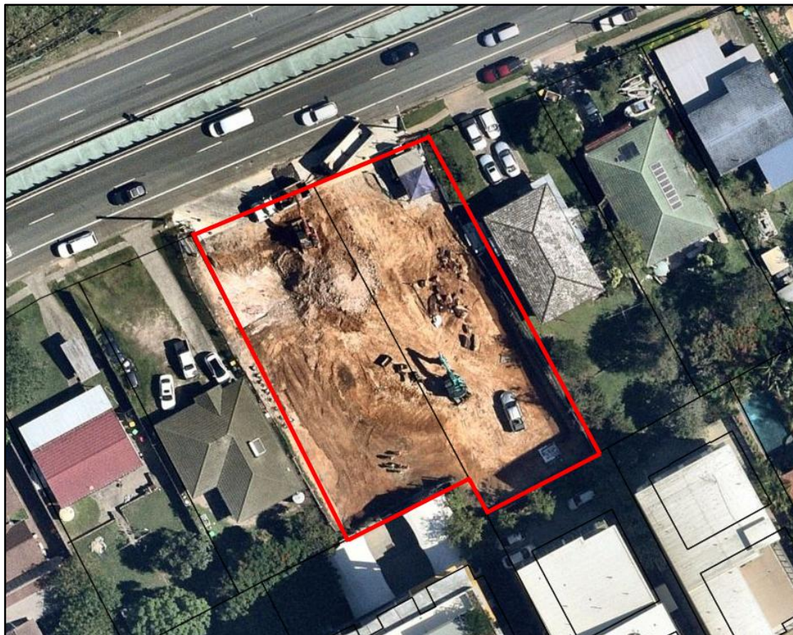
Figure 1: Subject Site Aerial (Source: NearMap, image dated 3 December 2025)
