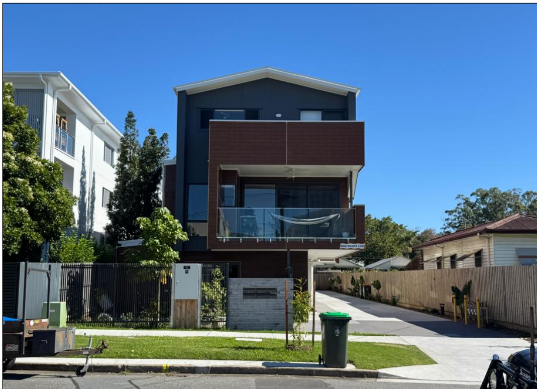
Figure 7: Site Photograph. Adjoining neighbour at 22 University Road, Mitchelton as viewed from the University Road frontage.
