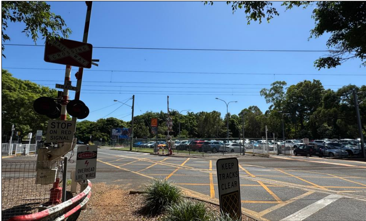
Figure 8: Site Photograph. The Subject Site is located within 250m walking distance of the public pedestrian access point to the Mitchelton Train Station.
