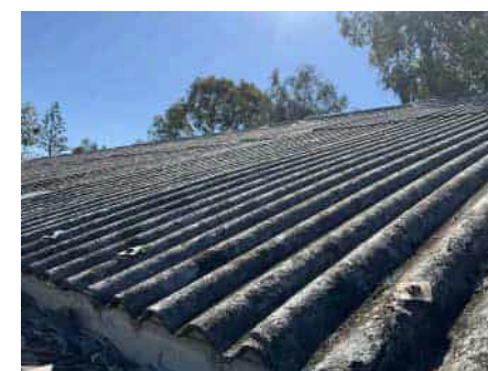
Roof sheeting - Overview
