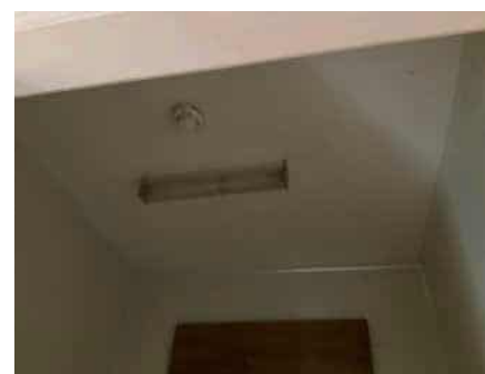
Women's toilet ceiling
