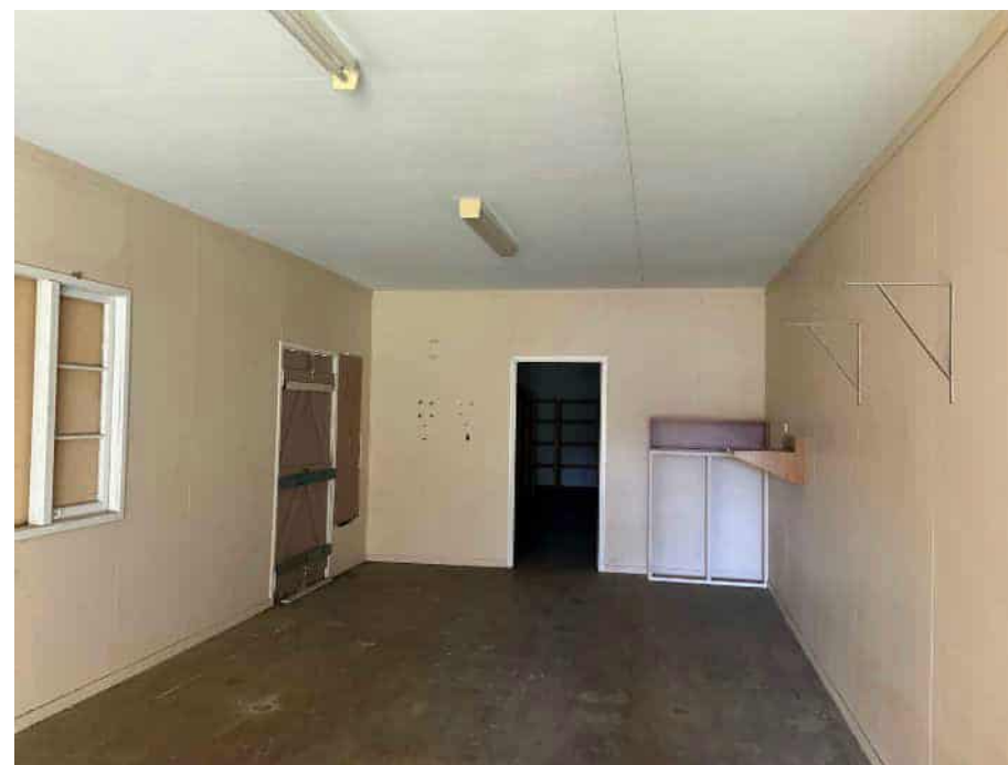
Northwest room walls
