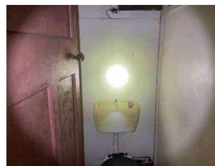
Infill panels behind toilets
