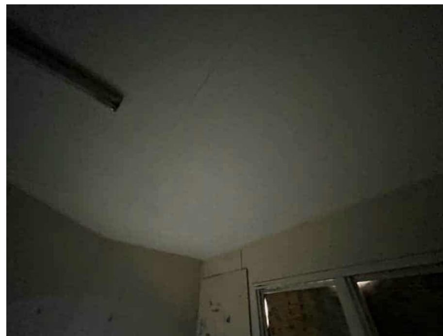
Main room ceiling
