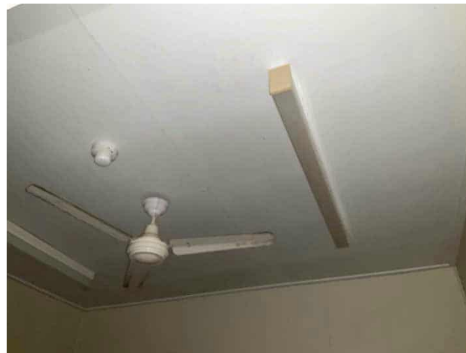
East rooms ceiling
