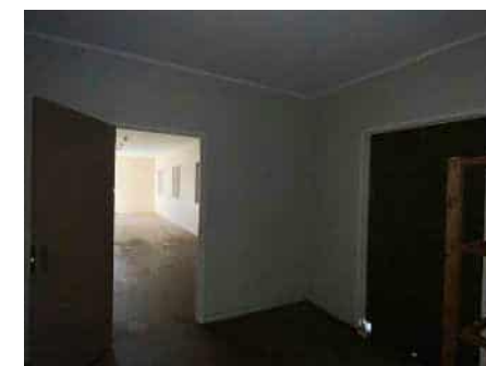
Northeast long room walls
