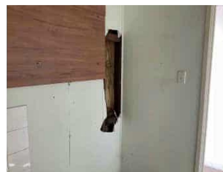
Male toilet walls
