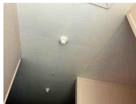
Entry foyer ceiling lining
