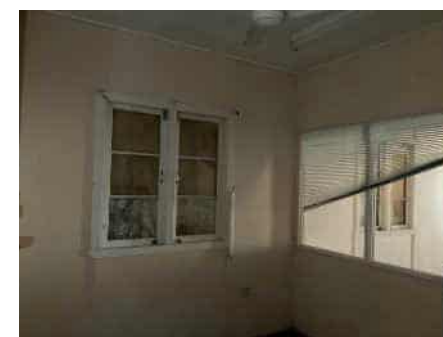
East rooms walls
