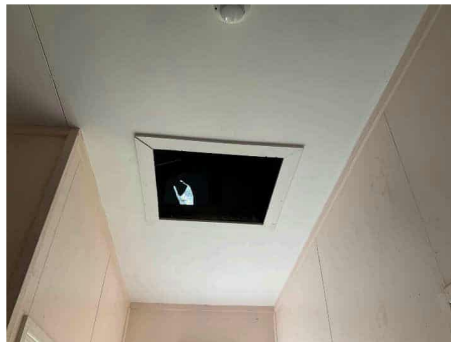
Entry foyer ceiling lining
