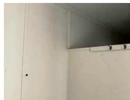
Shower room walls
