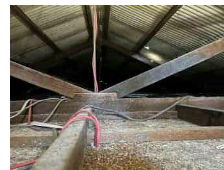
Roof void overview
