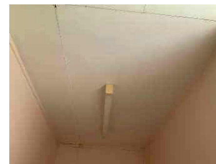
Entry foyer ceiling lining
