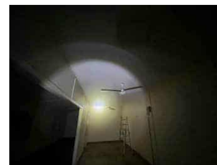
Main room ceiling
