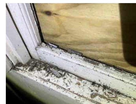
South rooms window putty
