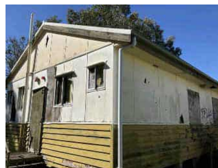
Wall and gable cladding - Overview
