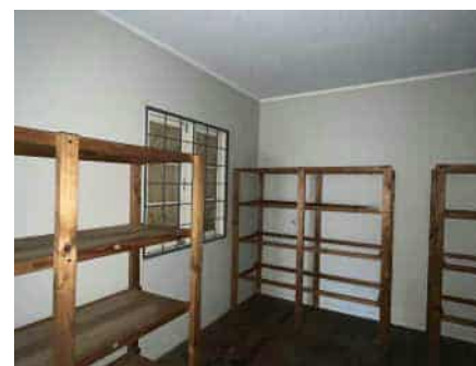
Northeast long room walls
