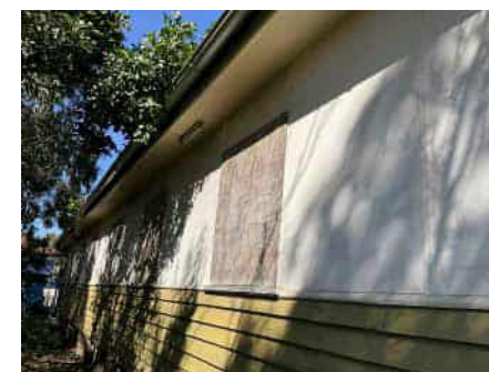
Wall and gable cladding - Overview
