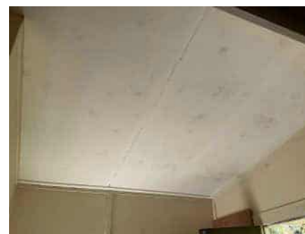
Southwest entry ceiling
