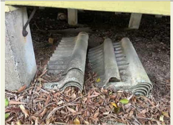
Figure 8-5: Disused ACM roofing material below building
