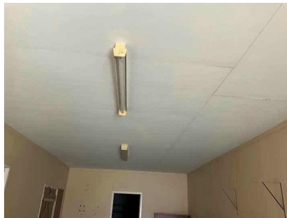
Northwest room ceiling
