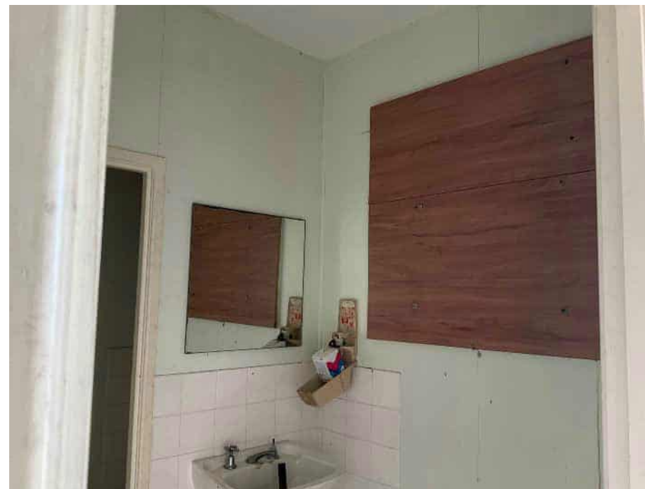
Male toilet walls
