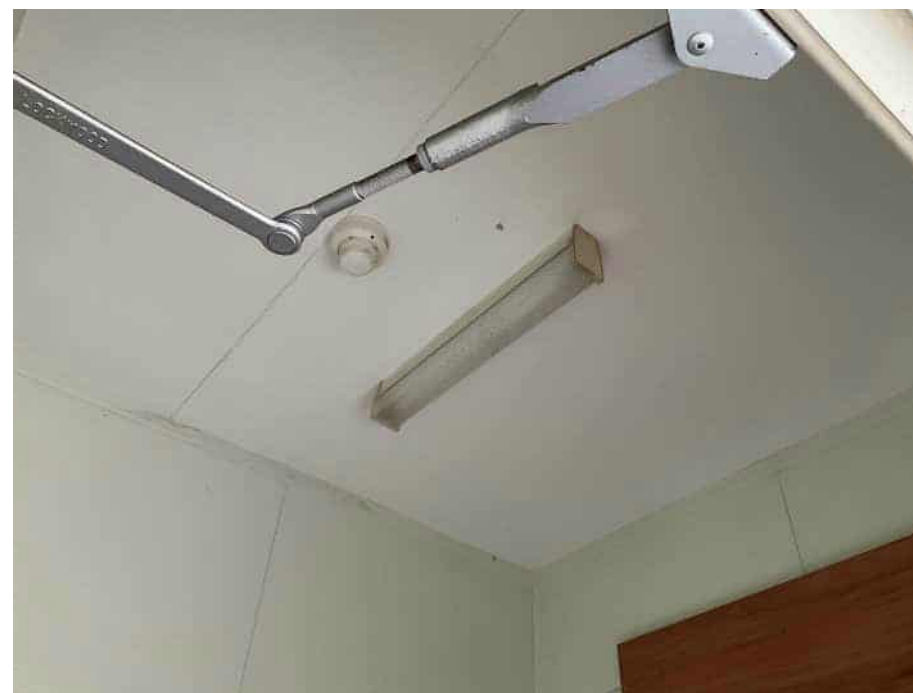
Male toilet ceiling lining
