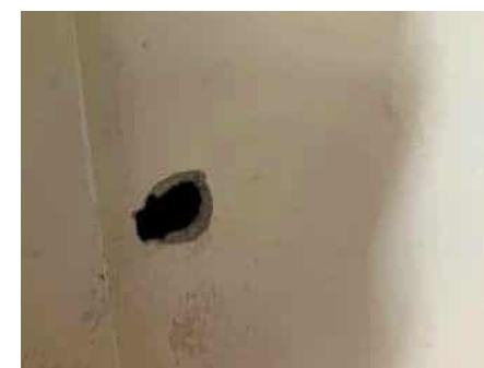
Shower room walls
