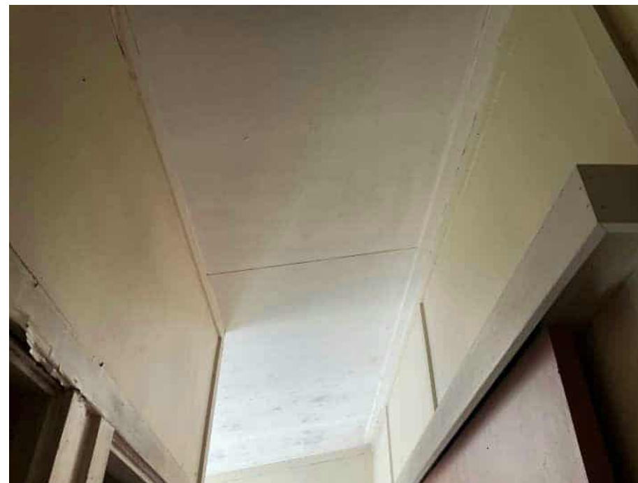
Southwest entry ceiling
