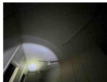
Main room ceiling
