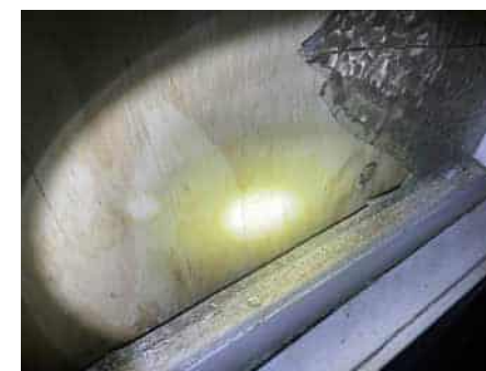
Windows with window putty
