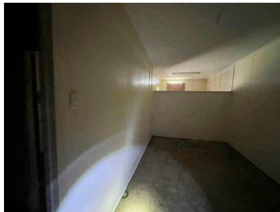
Secondary room wall lining
