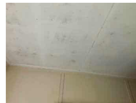
Southwest entry ceiling
