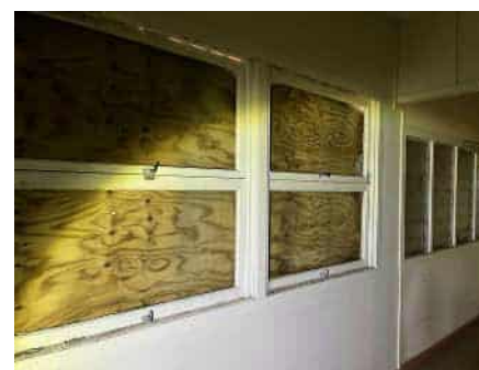
South rooms window putty
