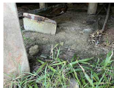
Debris below building
