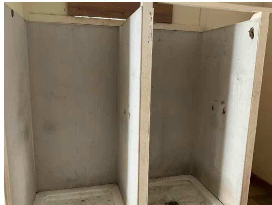
Shower room cubicle partitions
