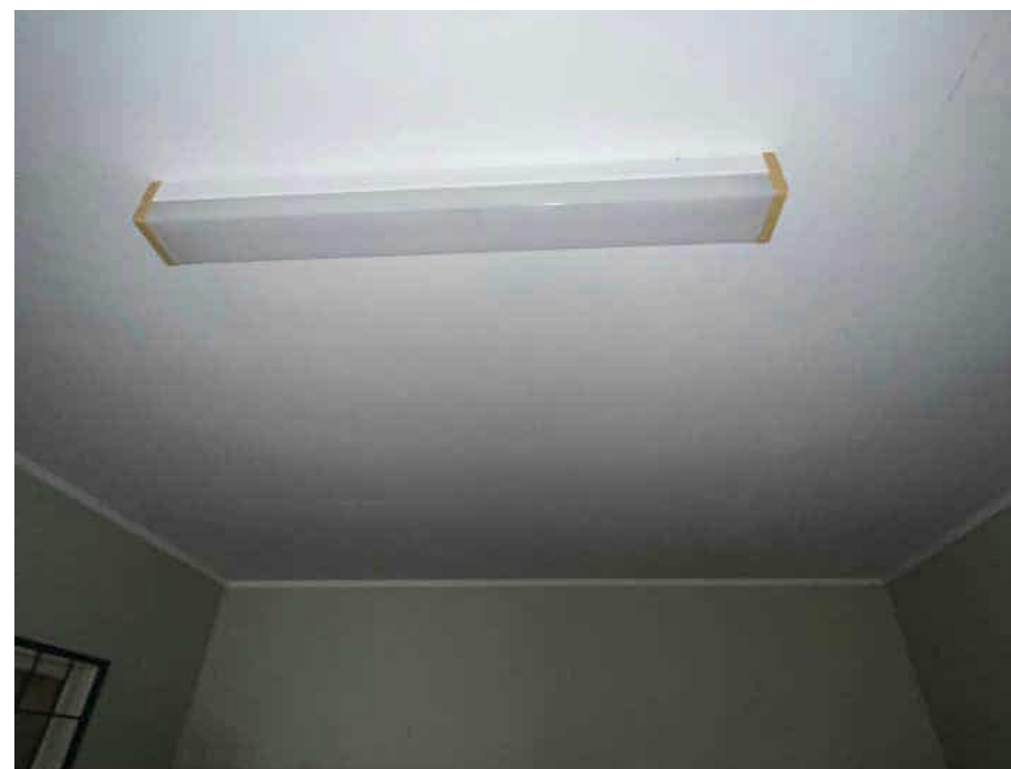
Northeast long room ceiling
