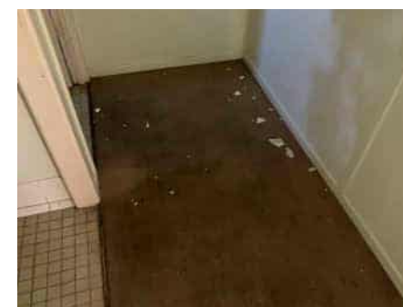
Floor where FC subfloor extends below vinyl
