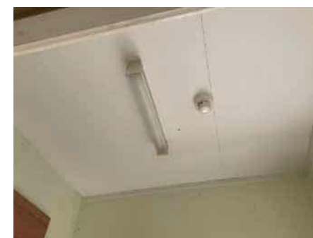
Male toilet ceiling lining
