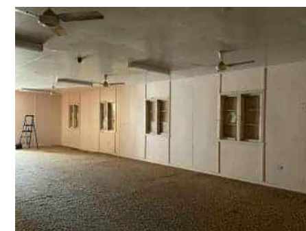
Main hall walls
