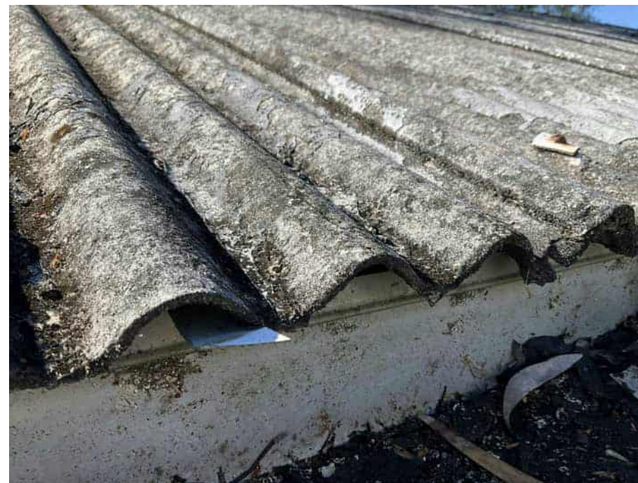
Roof sheeting - Overview
