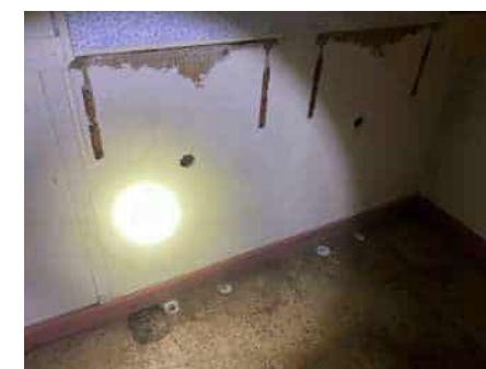
Infill panels below removed sink
