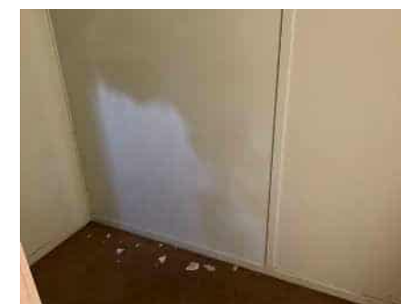
Women's toilet walls
