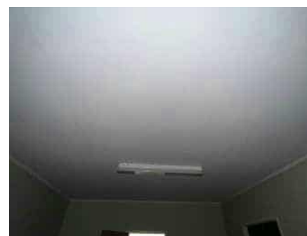
Northeast long room ceiling
