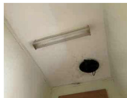
Male toilet ceiling lining
