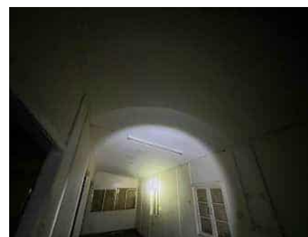
Enclosed sunroom ceiling
