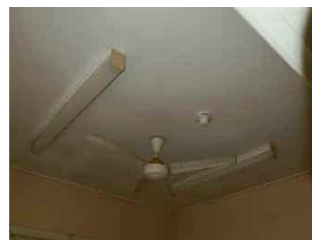
East rooms ceiling
