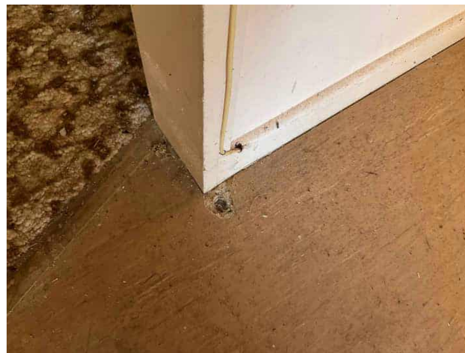
Floor where FC subfloor extends below vinyl
