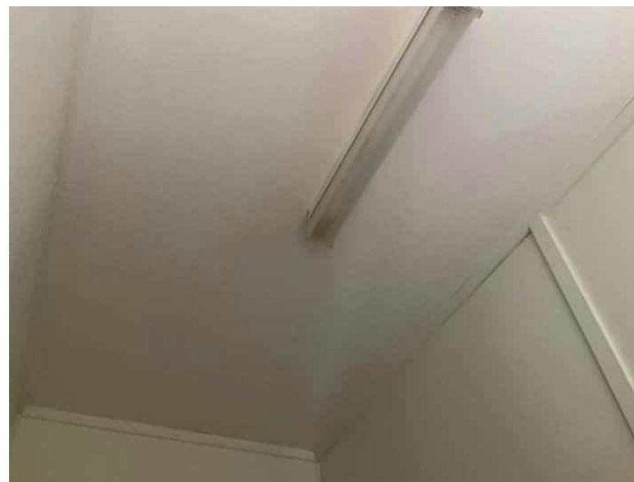
Women's toilet ceiling
