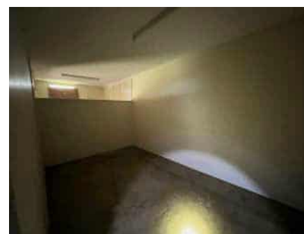
Secondary room wall lining
