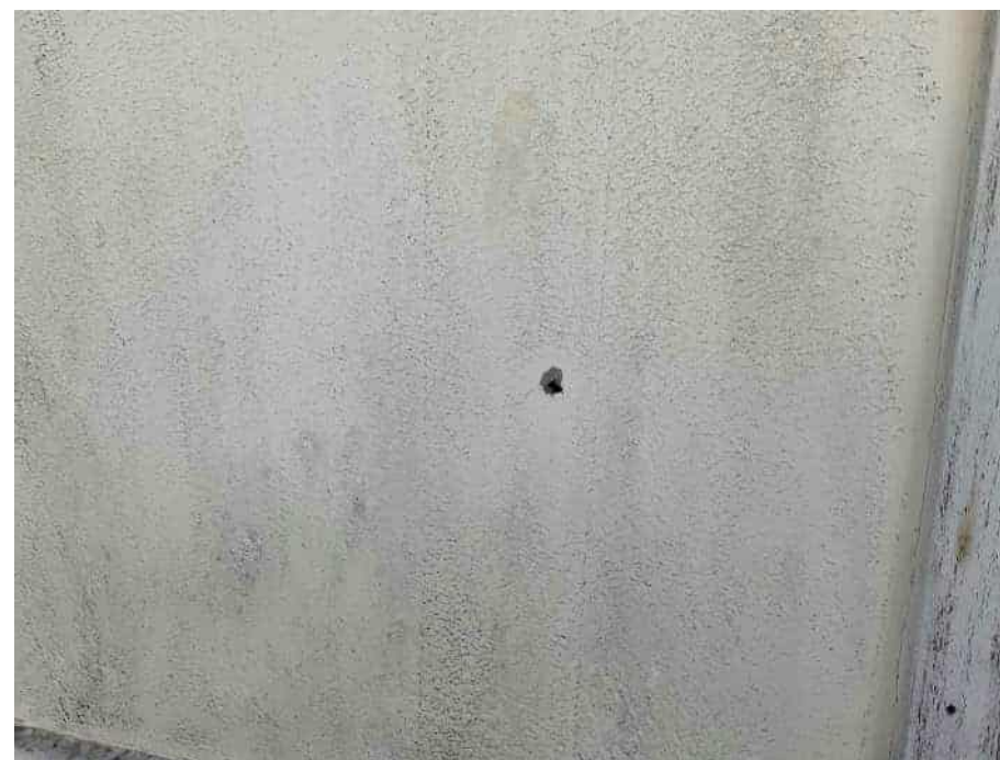
Sample location of wall cladding
