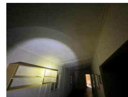
Enclosed sunroom ceiling
