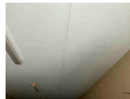
Northwest room ceiling
