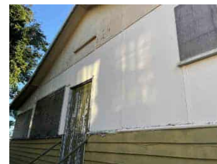
External cladding overview
