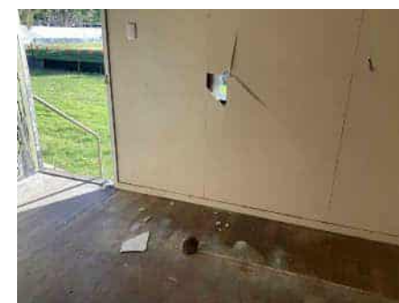
Northwest room walls
