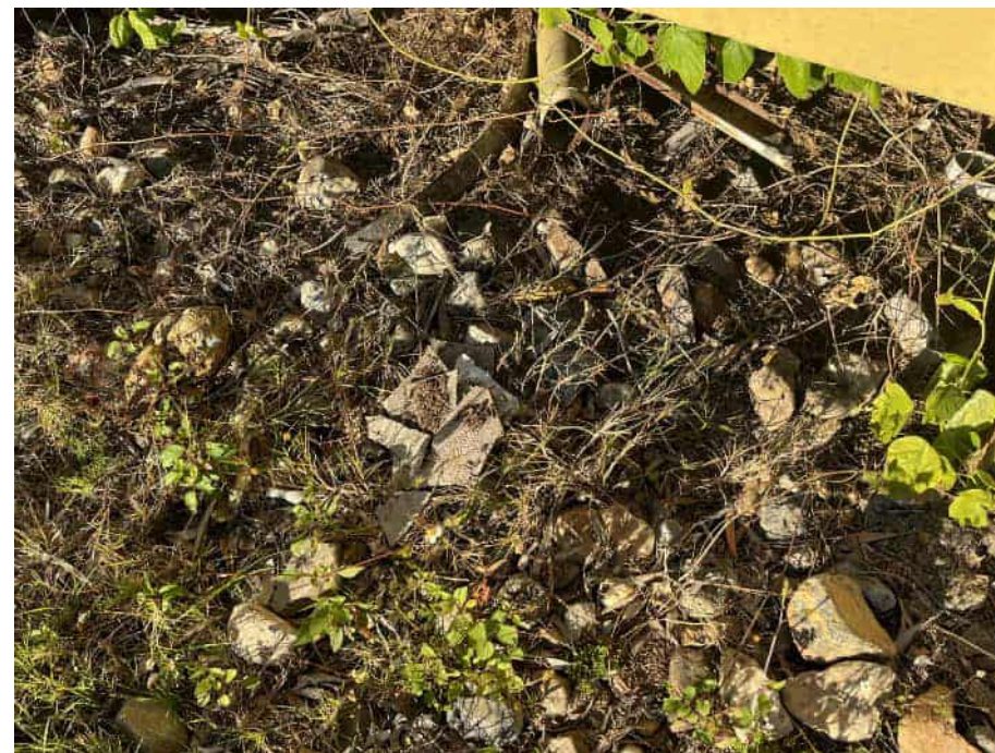
Debris on ground
