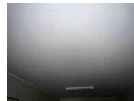
Northeast long room ceiling
