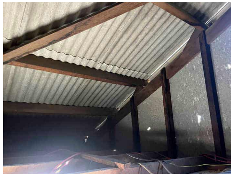
Roof void overview
