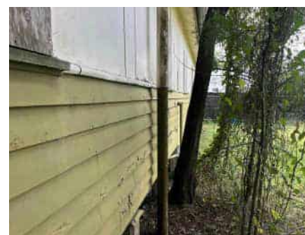
Waste vent pipe on south elevation
