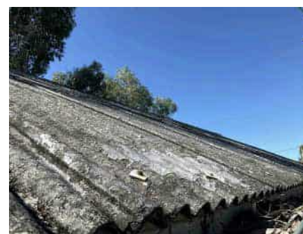
Roof sheeting - Overview
