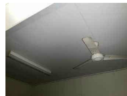
East rooms ceiling
