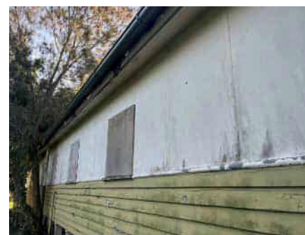
External cladding overview
