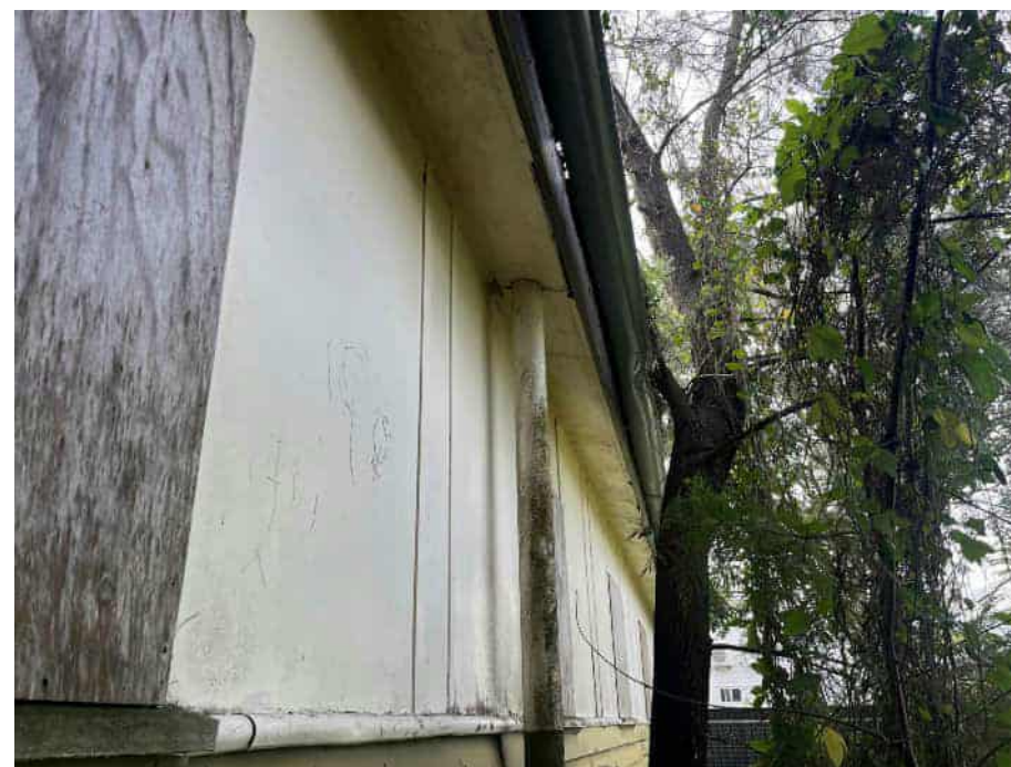
Waste vent pipe on south elevation
