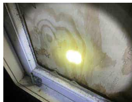
Windows with window putty
