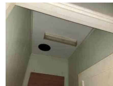
Women's toilet ceiling
