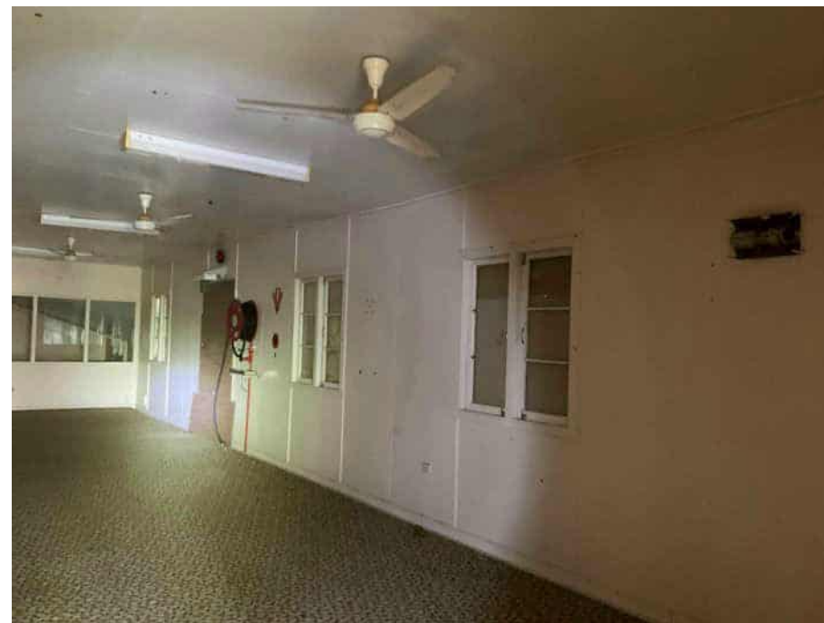
Windows with window putty
