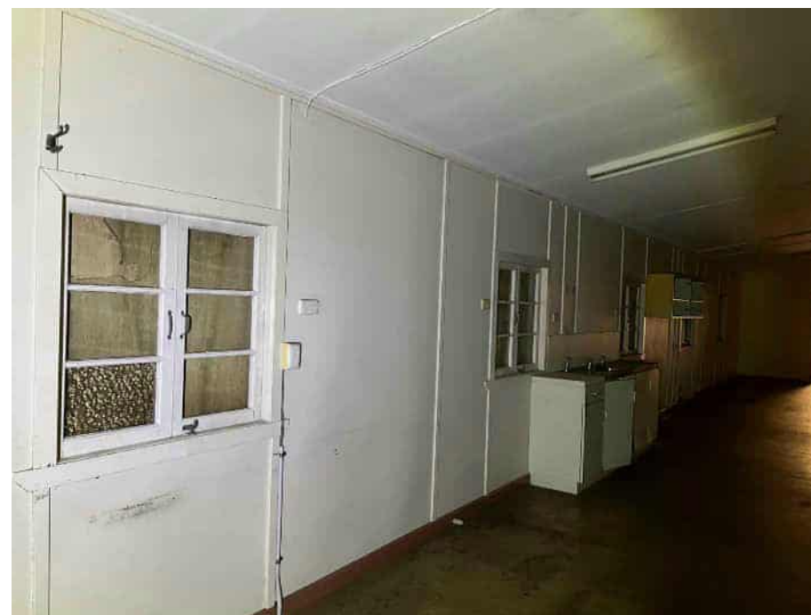
Enclosed sunroom ceiling
