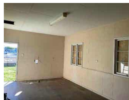
Northwest room walls
