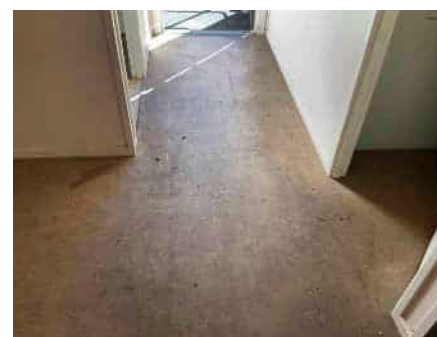
Floor where FC subfloor extends below vinyl
