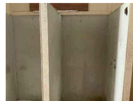
Shower room cubicle partitions
