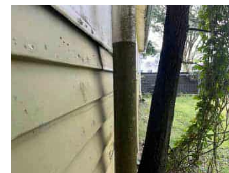
Waste vent pipe on south elevation
