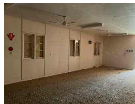
Main hall walls
