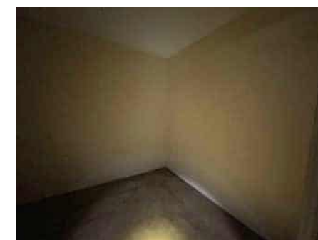
Secondary room wall lining
