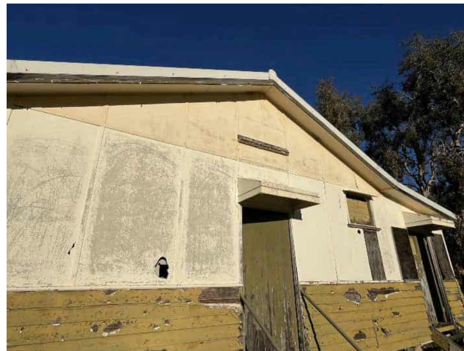
External cladding overview
