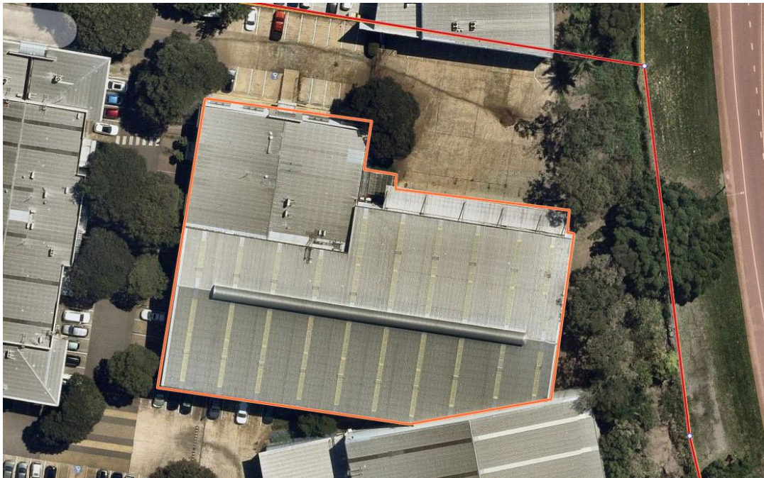
Figure 7: Aerial of the existing warehouse ( Source: Nearmap, 2026)
