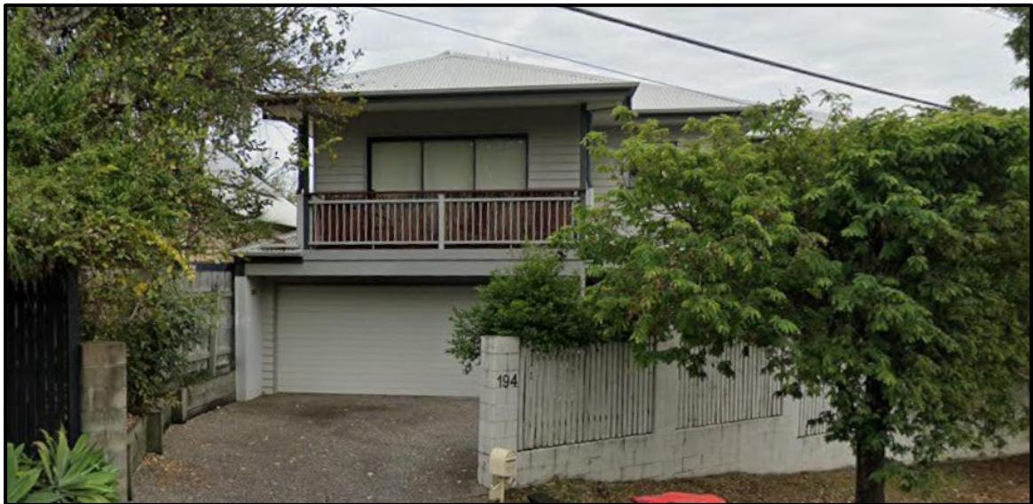
194 Windsor Road – Google Street View Post-1946 house
