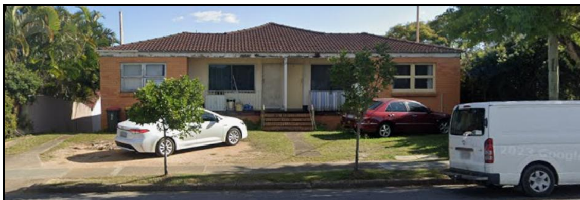
116 Windsor Road – Google Street View Post-1946 building/structure
