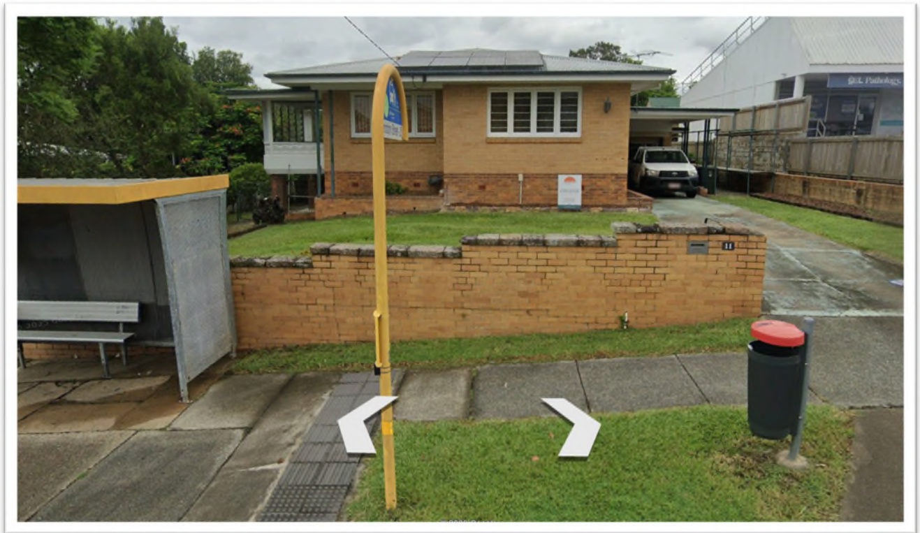
Site Photo 1: View of 11 Ekibin Road, Annerley from the street frontage
