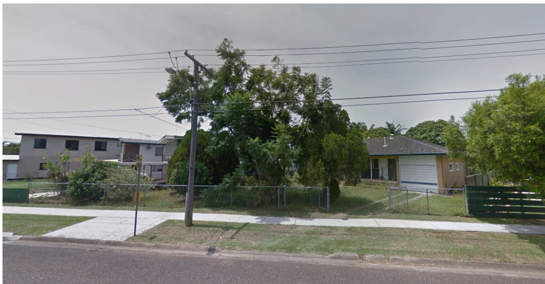
View of street frontage prior to demolition
