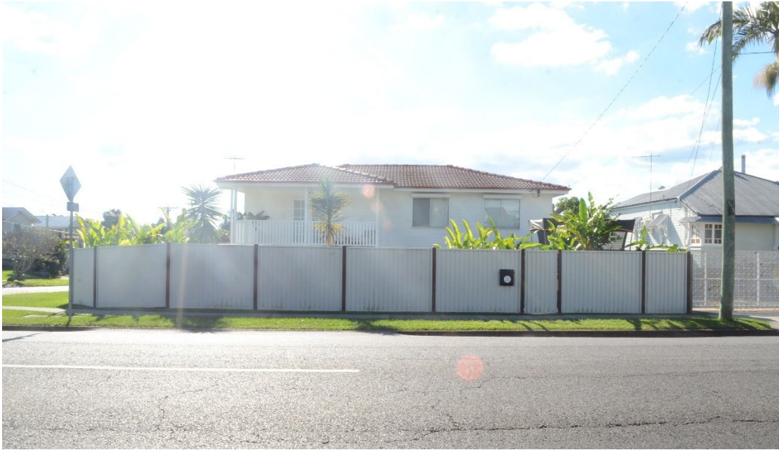
View towards 1 French Street, opposite the subject site to the north.
