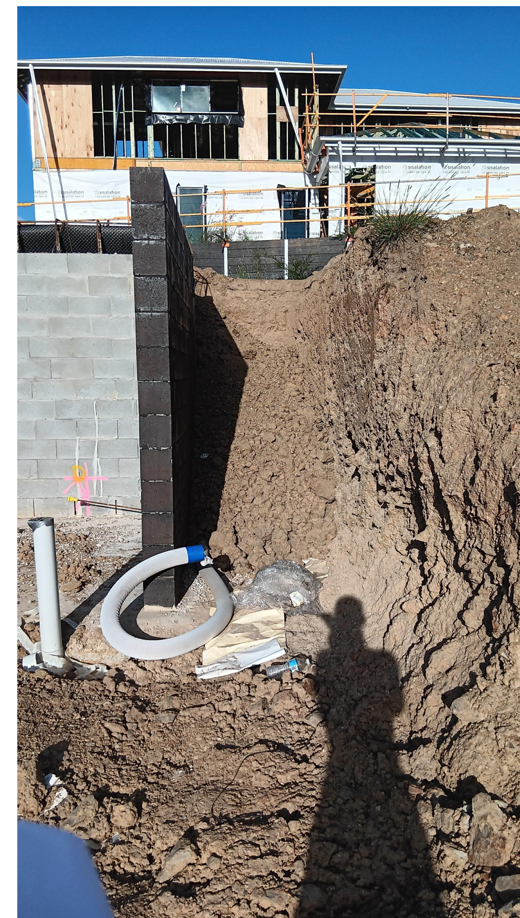
60 Halifax Street to 62 Halifax Street which requires shoring
