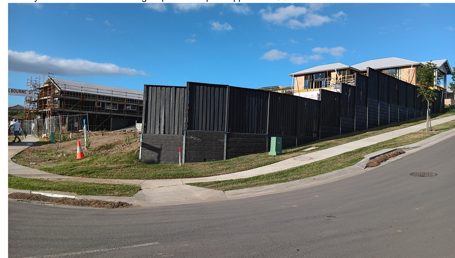
Photo from Holbourne Street looking at large retainer wall and fencing to 62 Halifax Street
