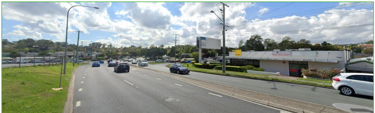
Figure 14 – District Centre along Moggill Road and Marshall Lane (Source: Google Maps)
