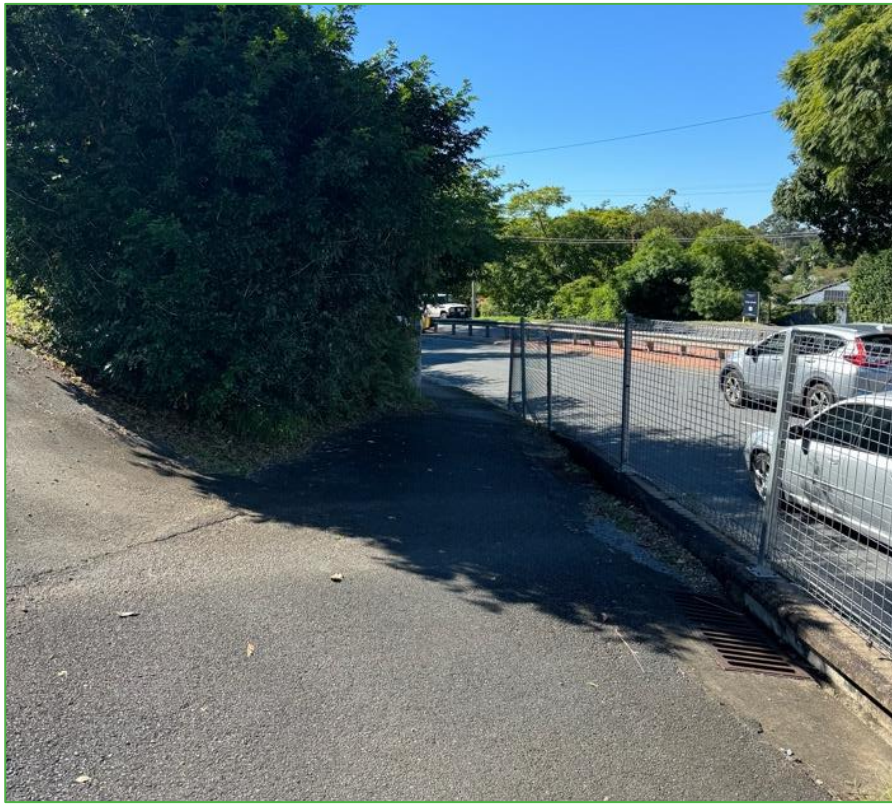
Figure 7 – Existing verge at the frontage of the site (Source: Gilvear Planning site visit 22 May)
