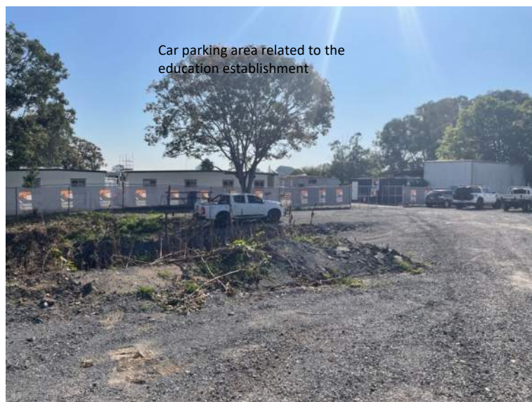
Figure 6 – Car parking area for the educational establishment (source: ARC Planning)
