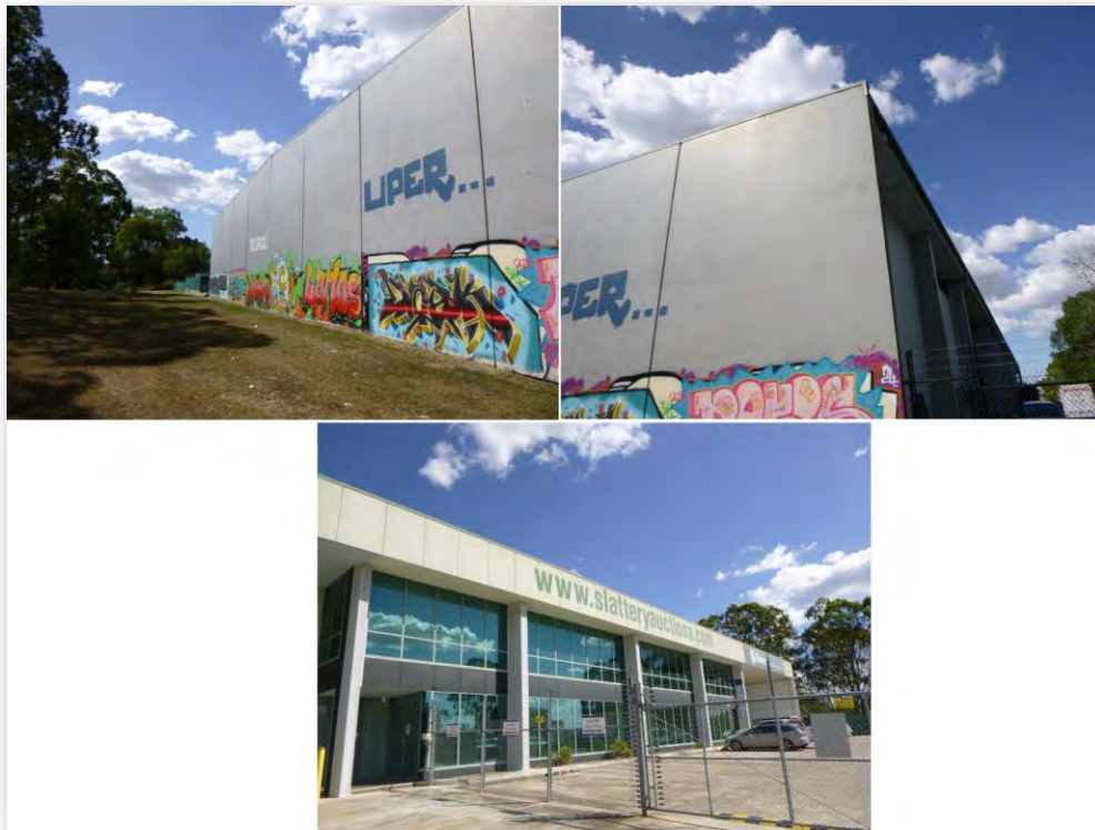
Figure 12. The gymnasium will be a building within a building, complying with BAL 12.5 of AS3959
