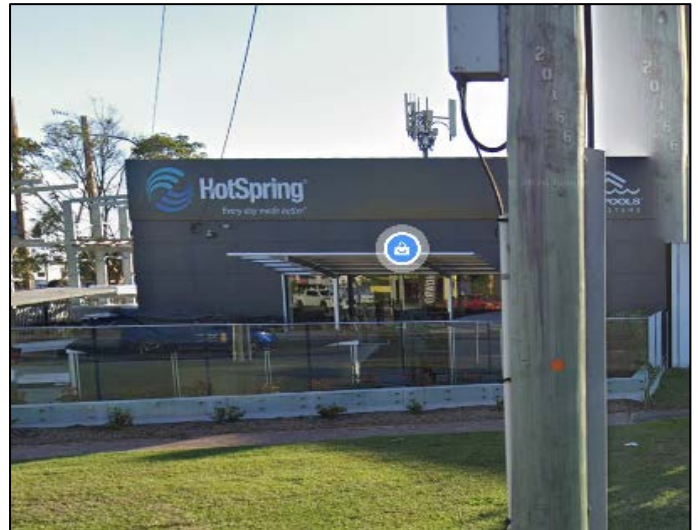
Photo 2: Adjoining Property – 819 Beaudesert Road, Archerfield
