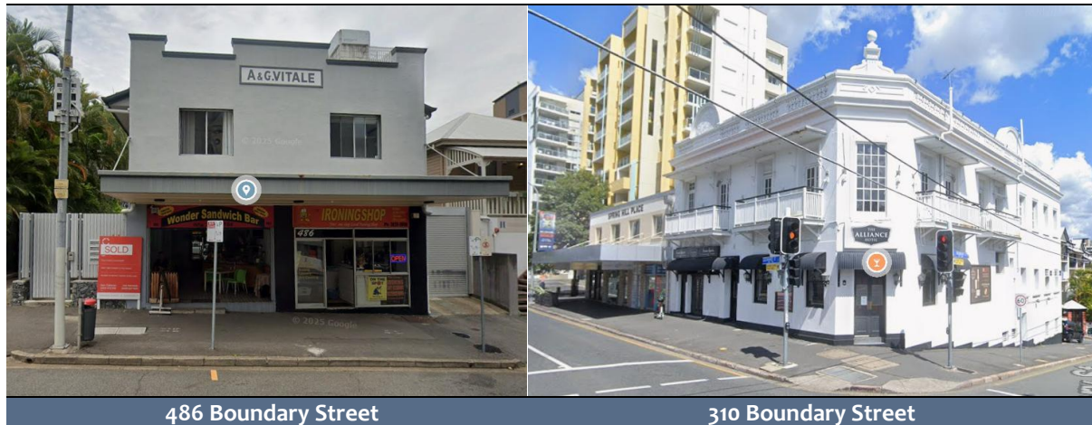
Figure 2 – Nearby examples of Art deco architecture
