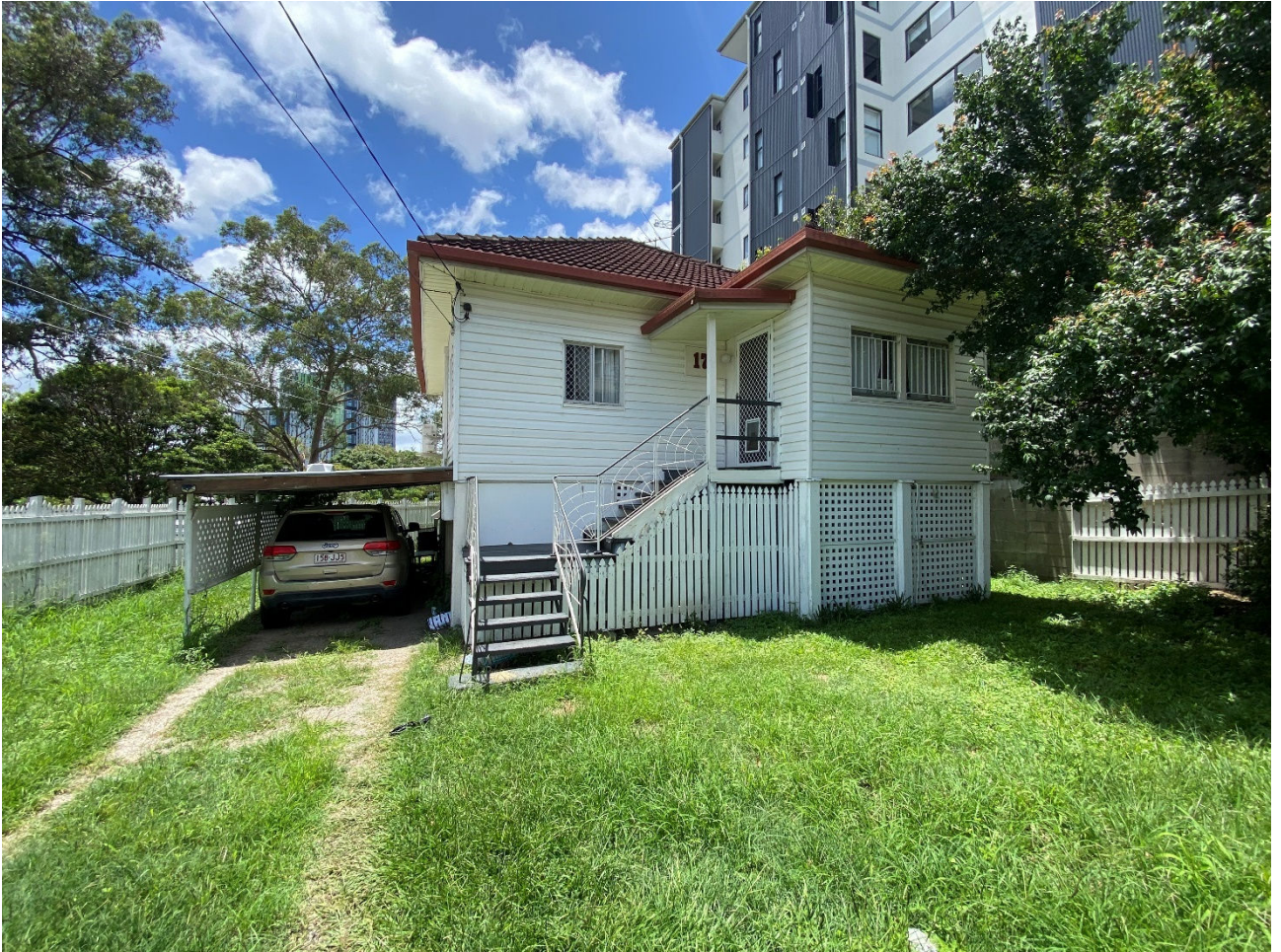
Photograph 1 – Existing site condition (looking north)
