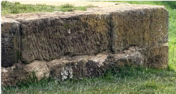
INDICATIVE SANDSTONE CHIMNEY FOUNDATIONS
