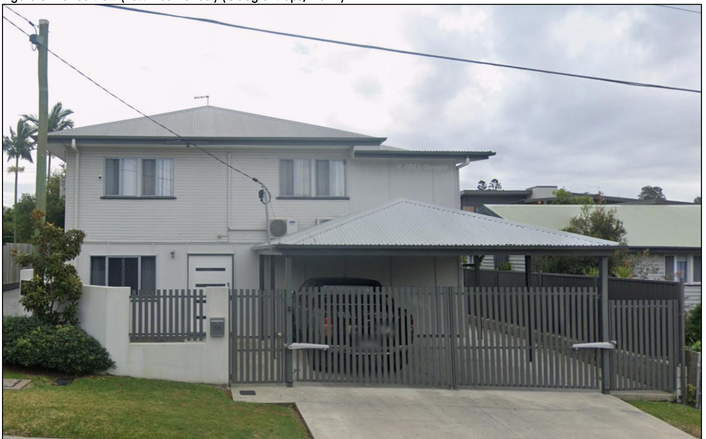
Figure 3 – Streetview (Rawlinson Street) (Google Maps, 2021)
