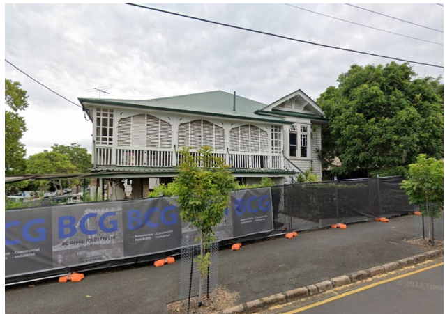
Picture 4 – Local Heritage Place at 469 Bowen Terrace
