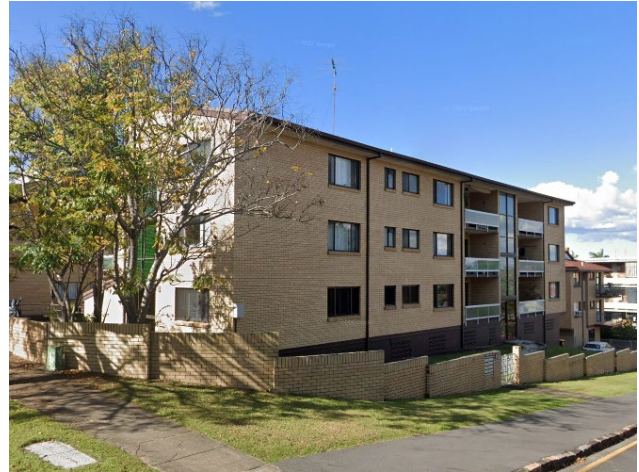
Picture 2 – 3-4 storey apartment building at 16 Moreton Street, located to the east of the site.
