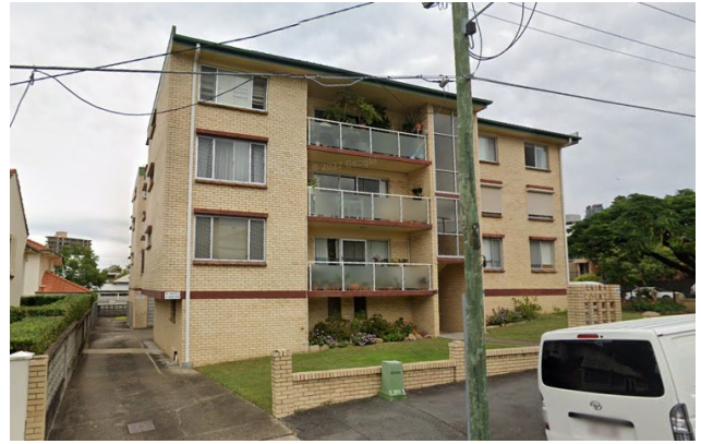
Picture 6 – 4 storey Multiple Dwelling south-west of the site at 439 Bowen Terrace
