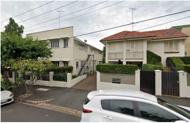
Picture 5 – Multiple dwelling and dwelling house located to the south of the site at 453 & 443 Bowen Terrace
