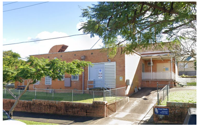
Picture 8 – Decommissioned Telstra Exchange Building opposite site to the north-west (corner of Bowen Terrace and Langshaw Street)
