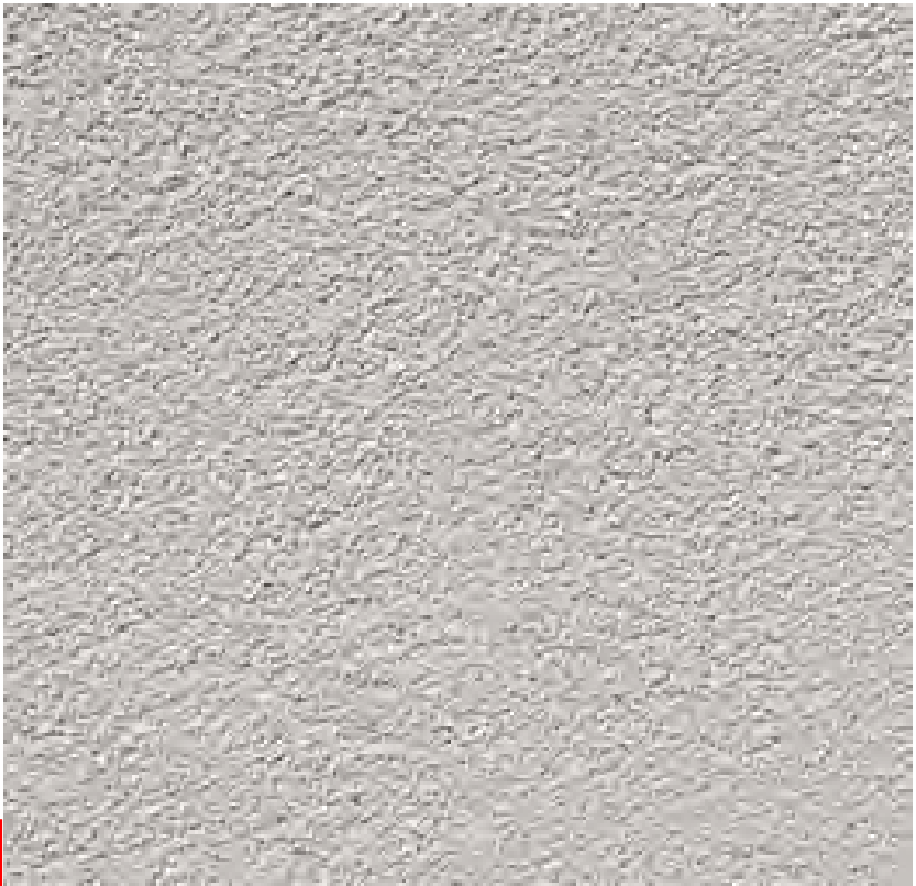
ROUGH ACRYLIC RENDERING (TEXTURED) TO ALL RENDERED EXTRIOR WALLS. COLOUR TO MATCH 'PT#' COLOUR CODES.
