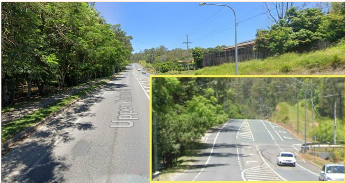
Figure 7-6 Eastbound Approach Sight Distance to Proposed Intersection
