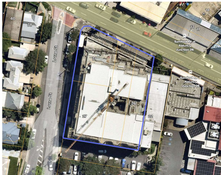
Figure 1 – Aerial Photo of Subject Site (dated March 2026) – demonstrating construction works onsite (Source: NearMap, 2026)
