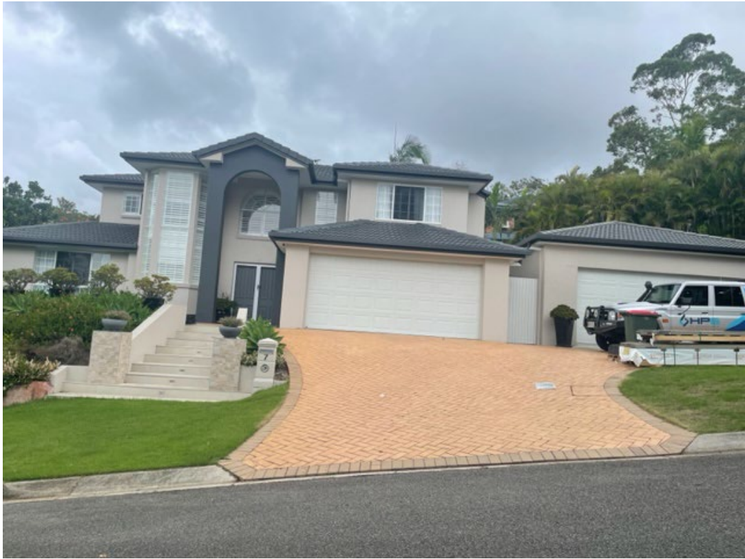
Photo 1: Subject property – Viewed from frontage
