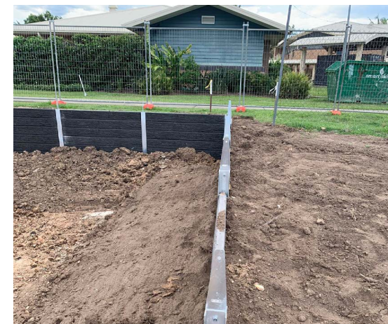
RETAINING WALLS AROUND SITE BOUNDARY
