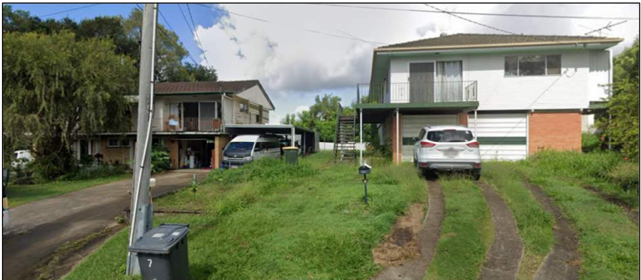
Figure 4. Existing Northern Façade (Google Maps, 2024)
