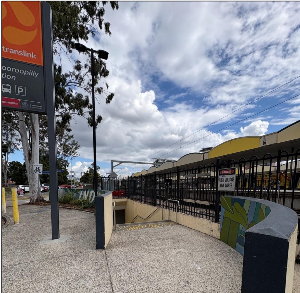
Figure 7: Entrance to Indooroopilly Railway Station
