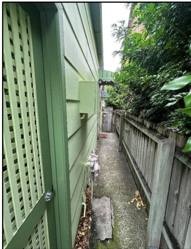
Photo of the north-west side of the house – Heritage impact report, Andrew Ladlay Architect
