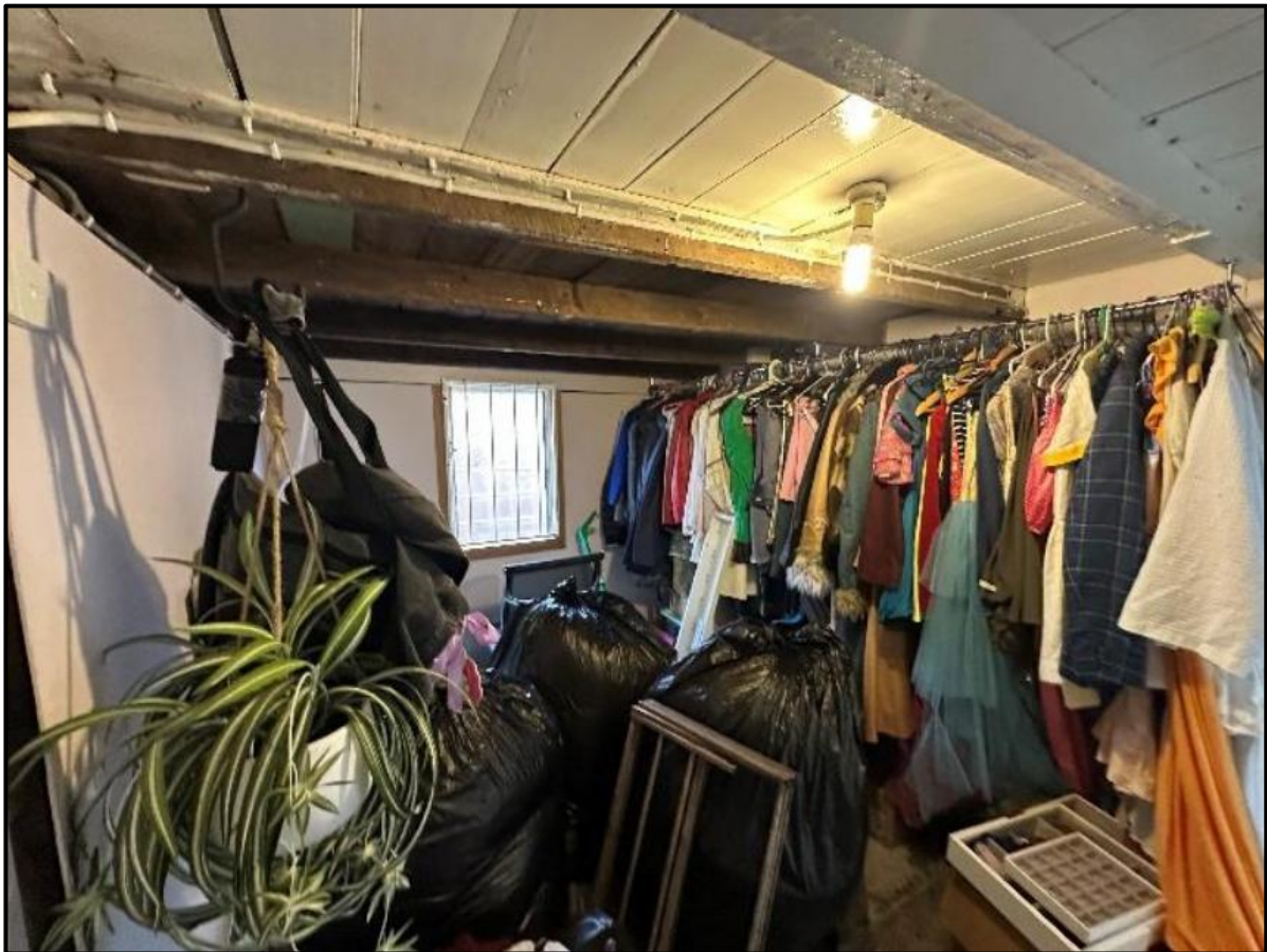
Photo of the undercroft space of the house – Heritage impact report, Andrew Ladlay Architect
