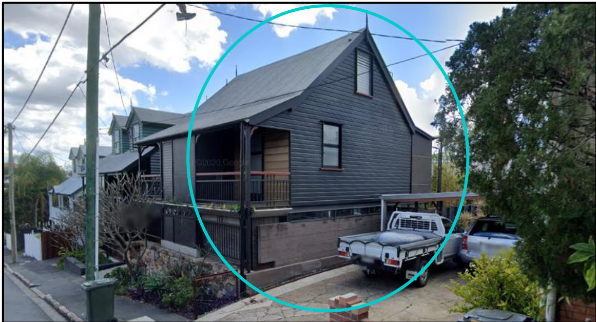
11 Isaac Street – Google Street View Photo showing the existing house is built in close proximity to the side boundary
