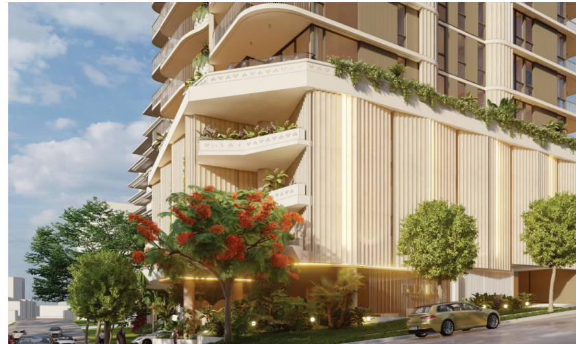
North west corner / western façade - Jephson Street
