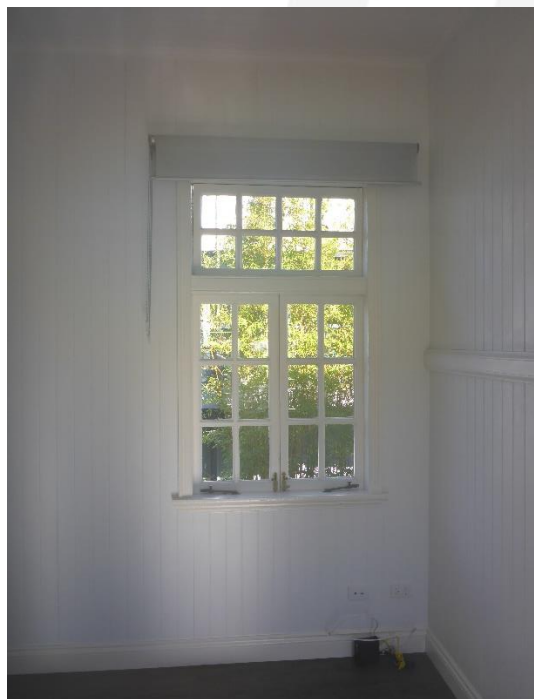
Figure 28: An interior view from within the living space of Unit 6 showing the original window assembly within the southern side wall – also refer to Figure 6 (above), intact interior wall construction etc. (Source: VAULT)
