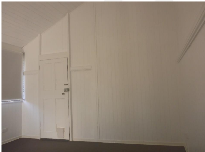
Figure 50: An interior view of the bedroom space of Unit 1, which is set within an enclosed verandah space at the front of the heritage building. The raked and timbered soffit of the verandah roofline is visible at image top left. (Source: VAULT)
