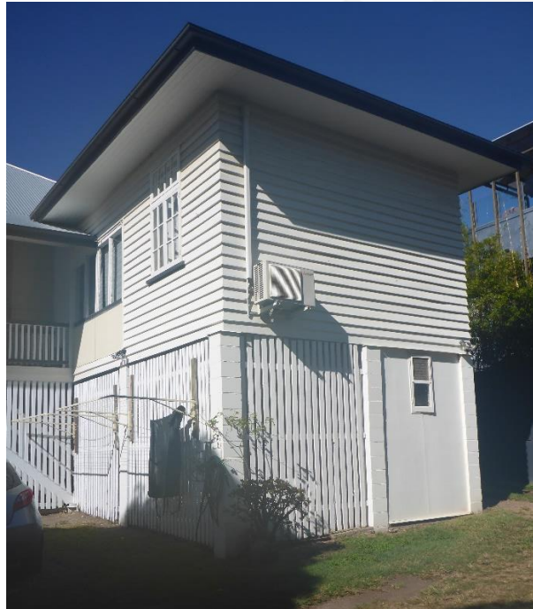
Figure 9: An oblique view of the rear wing projection of the subject heritage residential building, which originally comprised the Kitchen wing of “Mimosa” connected to the core of the residence by an open verandah. (Source: VAULT)
