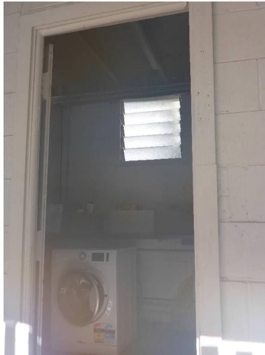
Figure 73: A more detailed view of the entrance into the undercroft level laundry enclosure showing the modern door and glass louvres that have been integrated into this subsequent addition set beneath the heritage building. (Source: VAULT)
