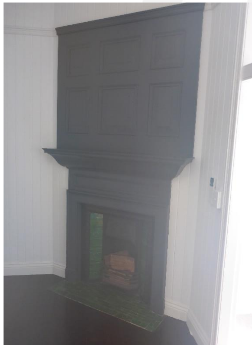
Figure 42: A detailed view of the corner fireplace assembly with Unit 1 that remains as an intact, original feature of the “Mimosa” residence. (Source: VAULT)
