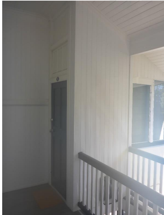
Figure 19: Another view from within the rear verandah space, which shows the VJ-panelled enclosure at the rear corner of the verandah with a doorway integrated into same that leads into the rear wing of the building. (Source: VAULT)
