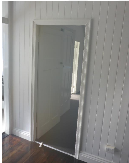
Figure 44: A detailed view of the doorway leading into the Bedroom of Unit 1, which is located at the front of the heritage building. (Source: VAULT)
