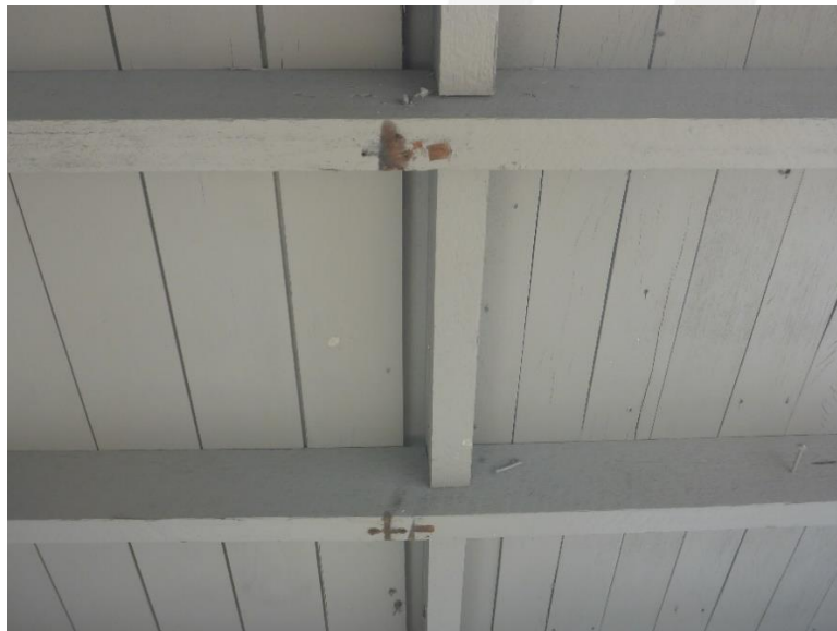
Figure 74: A more detailed view of the sub-floor framing (and associated floor linings) showing the differential in the gauge of the timber flooring lining what was the original core of the heritage residence, "Mimosa" (at image left) and the transition to narrower gauge decking boards (at image right) where the open side verandah space has been enclosed and integrated into the habitable areas of the building. (Source: VAULT)
