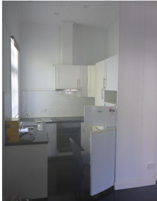
Figure 59: The kitchen alcove space within Unit 2 is clearly a contemporary kitchen joinery / plumbing installation set adjacent to an original window in the southern (side) elevation. (Source: VAULT)
