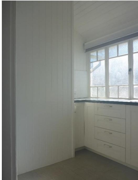
Figure 45: The contemporary kitchen installation set within the side verandah enclosure integrated into Unit 1 showing the raked and timbers soffit lining (at image top right) and the array of multi-paned, casement windows. (Source: VAULT)
