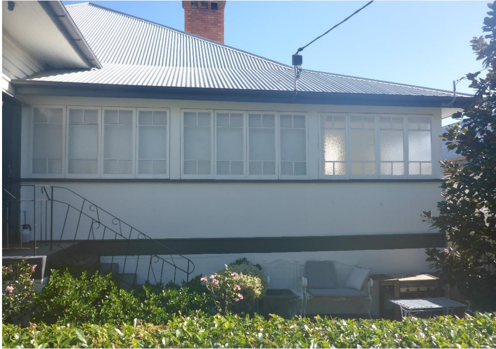
Figure 3: A more detailed view of the balance of the “Mimosa” street façade focused upon what was originally a wraparound verandah beneath a “broken back” roof line, which has now been fully enclosed. (Source: VAULT)
