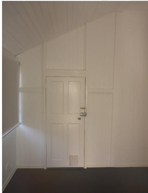
Figure 53: A more detailed view of the doorway from the bedroom space of Unit 1 into the vestibule space beyond at the front of the heritage building. The expressed framework set underneath the raked and timber ceiling serves to indicate the infill nature of this verandah enclosure while the framework visible at image right indicates the wall alignment of the original front wall of the “Mimosa” residence; now totally removed to amalgamate the adjoining spaces. (Source: VAULT)
