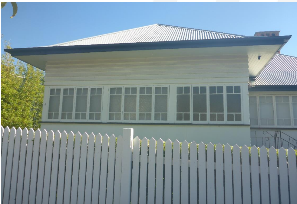
Figure 2: A more detailed view of the southern portion of the “Mimosa” street façade focused upon the projecting, hipped roof component of that façade, which originally comprised an open verandah (now enclosed). (Source: VAULT)
