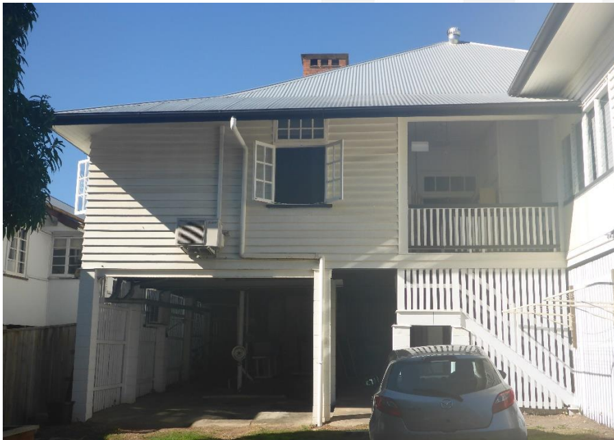
Figure 10: The balance of the rear elevation of the subject heritage residential building showing the rear verandah space and access staircase (at image right) and the rear wall of the house’s core with a hipped, “broken back” roof line over same. Also noted is the solid rear wall at image left, which was originally an open verandah return. (Source: VAULT)
