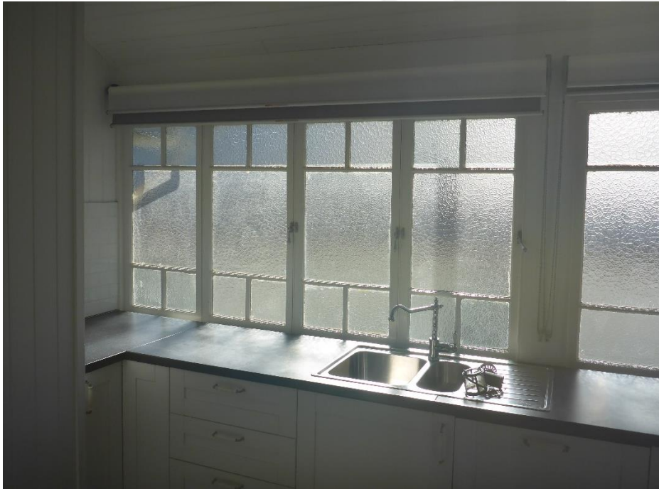
Figure 47: A more detailed view of the array of multi-paned casement windows that enclose the side verandah that now incorporates a contemporary kitchen installation for Unit 1 within same. (Source: VAULT)
