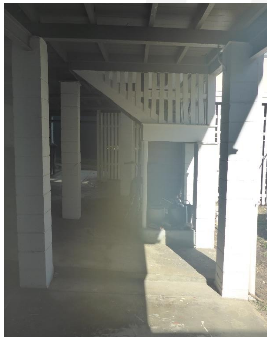
Figure 70: Another view through the extant undercroft space; this time proximate to the rear staircase and looking laterally across the rear portion of the building, which again shows the mixture of steel and concrete blockwork columns utilised as support structures beneath the heritage building. (Source: VAULT)
