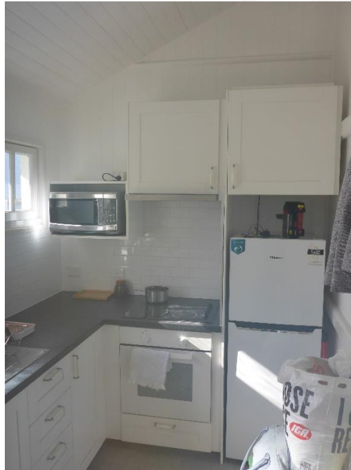
Figure 31: An interior view of the contemporary kitchen installation set within Unit 5 and showing the raked and timbered soffit lining that originally comprised part of a side verandah assembly. (Source: VAULT)
