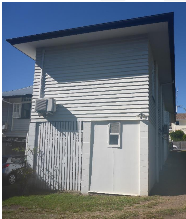
Figure 8: The western (rear) elevation of the subject heritage residential building, which comprises the remnant of the original Kitchen wing projecting behind the core of this building. (Source: VAULT)
