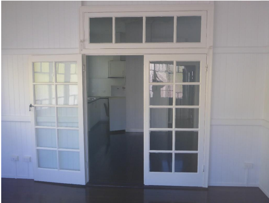
Figure 57: The view from the front bedroom space of Unit 2 looking through into the living space beyond (and contemporary kitchen installation in background). Note the multi-panes French doors and top light assembly set into what was the original front wall of the core of the “Mimosa” residence. (Source: VAULT)
