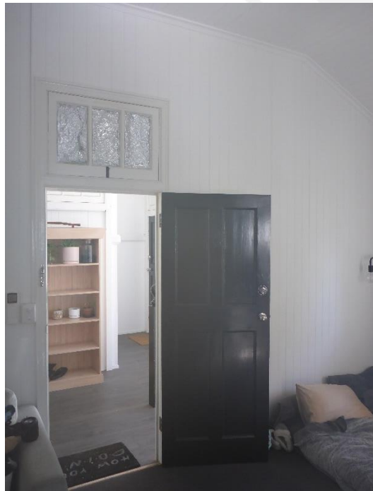
Figure 29: An interior view from within Unit 5 showing the original / intact door assembly (with top light panel over) and wall construction extant within that space and looking out onto the rear verandah space (in background). (Source: VAULT)
