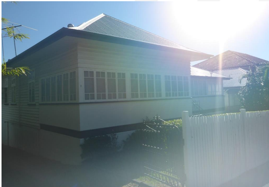
Figure 4: The reverse oblique street view of the subject heritage residential building, “Mimosa”, as viewed from the southern (front) corner of the subject site. This view reveals the stepped street façade and various “broken back” and hipped roof forms over. (Source: VAULT)
