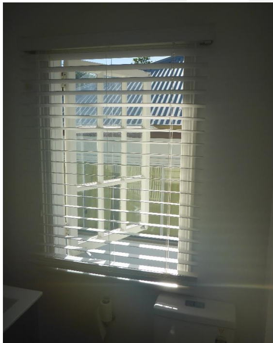
Figure 34: A detailed view of the original, multi-paned casement window within the bathroom space of Unit 5. (Source: VAULT)
