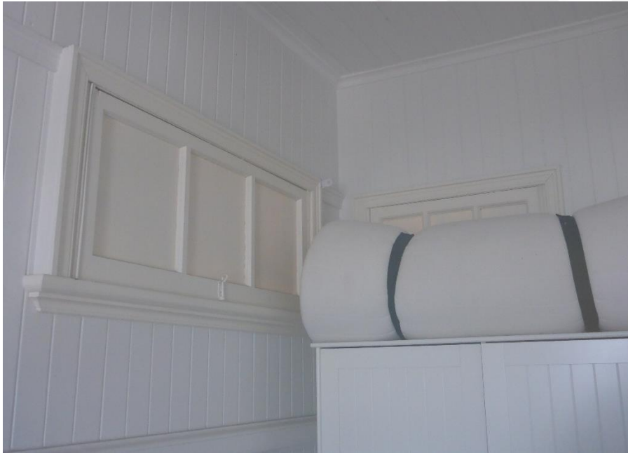
Figure 63: In the corner of the bedroom space within Unit 4, there are a pair of high-set, multi-paned awning windows that have now become internalised by later additions to the building. The glazing panels within both of these windows have subsequently been painted out for the privacy purposes. (Source: VAULT)
