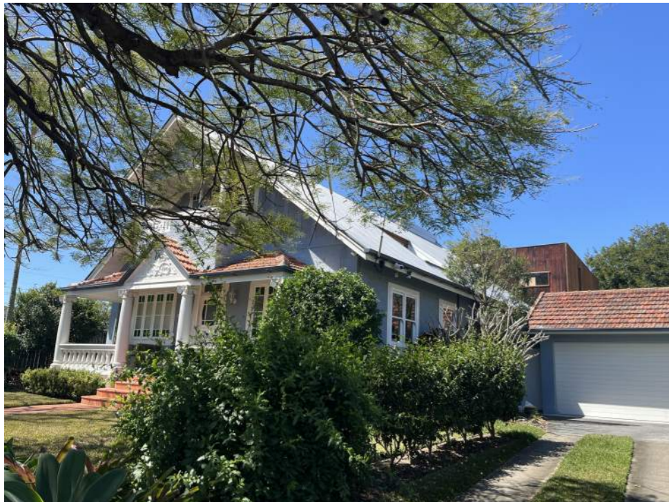
49 BULIMBA STREET - ON SITE CONDITION
