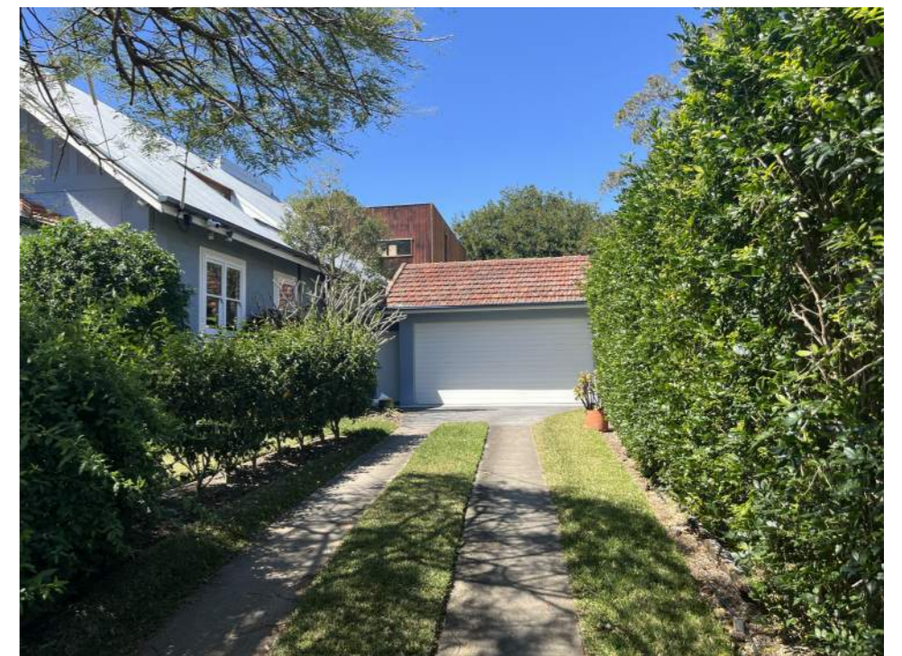
49 BULIMBA STREET - ON SITE CONDITION
