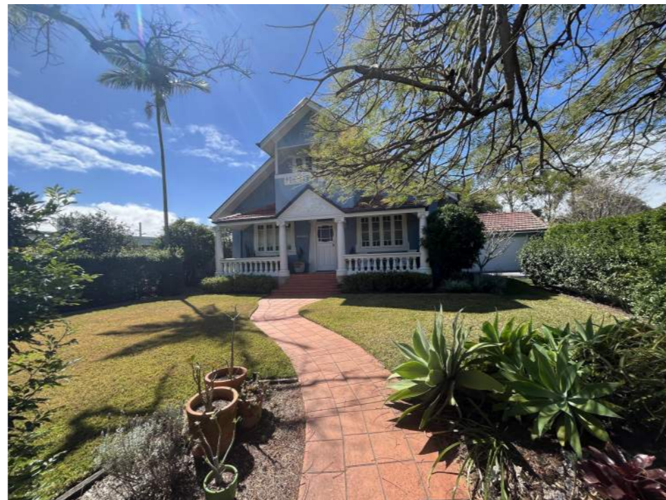
49 BULIMBA STREET - ON SITE CONDITION
