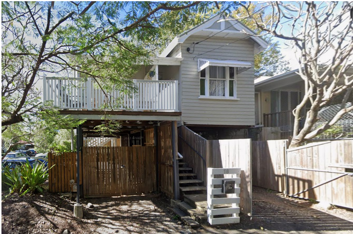
(Subject site – Google Streetview)
