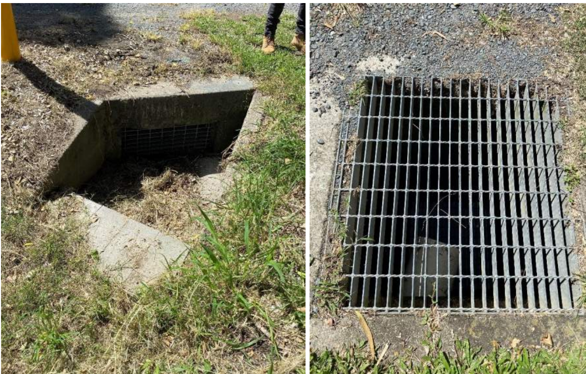
Figure 1.4 Drain 10 (left) and Drain 11 (right) – discharging runoff from non-operational areas
