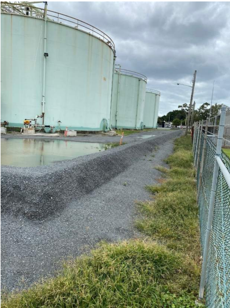
Figure 5.1 Bunding around operational areas in Drain 15 catchment
