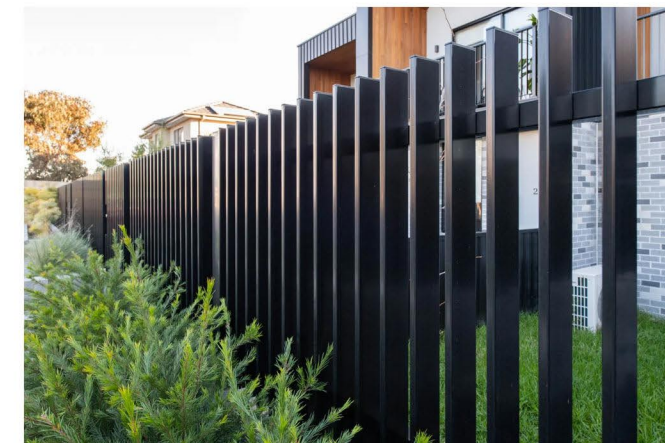
F1 01 INDICATIVE IMAGERY OF 1500mm HIGH ALUMINIUM BATTEN FENCE PAINTED BLACK (50% TRANSPARENCY) - WITH STEP DOWN WHERE REQUIRED. GATES TO MATCH
