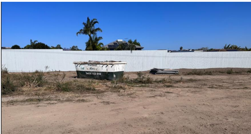
Figure 9 Constructed Acoustic Fence
