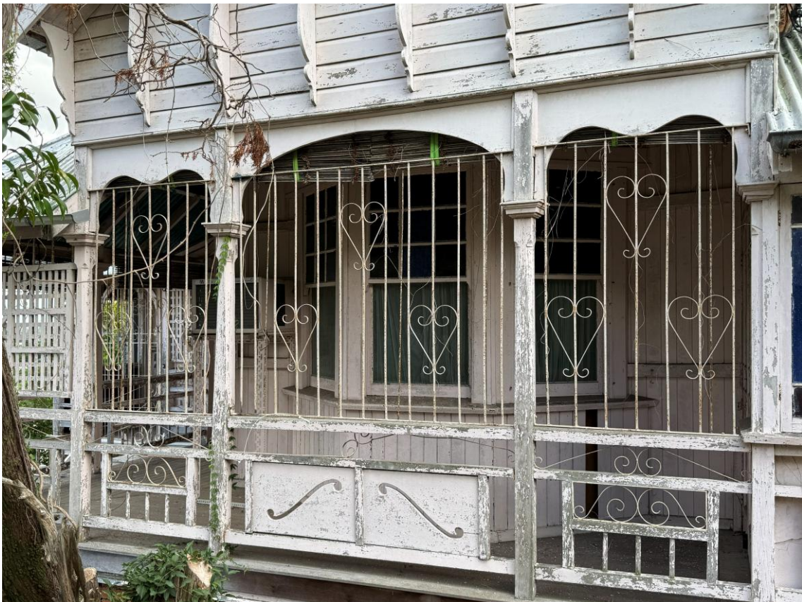
Figure 2: Perrot Street Frontage (2)
