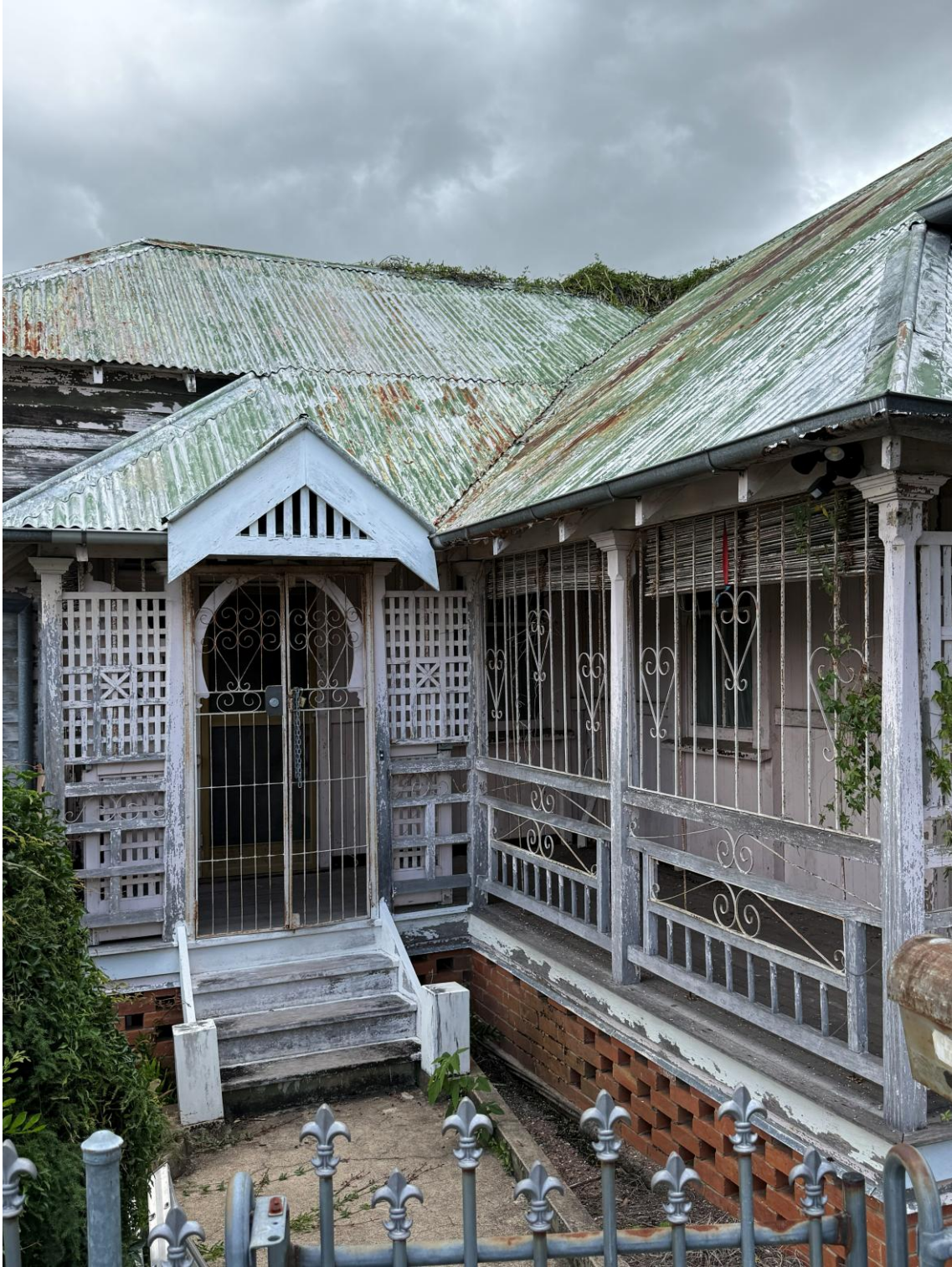
Figure 5: Perrot Street Frontage (5)
