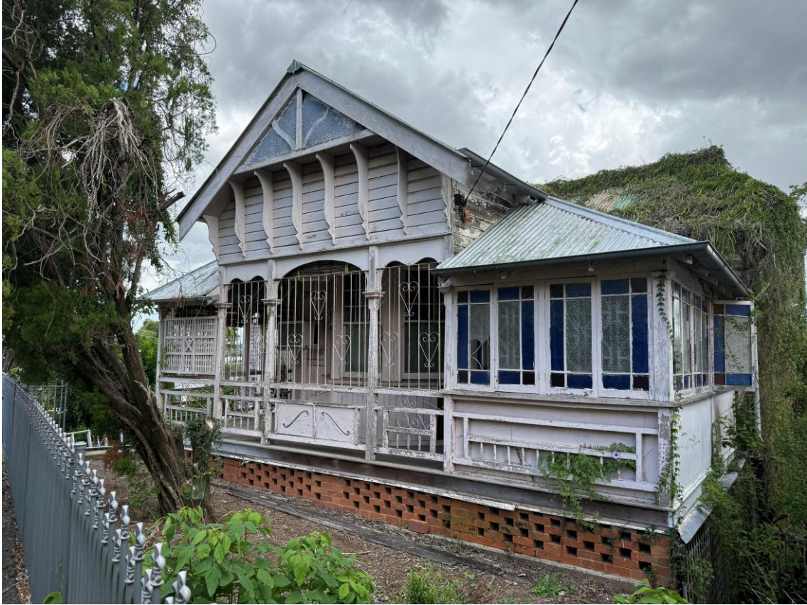
Figure 1: Perrot Street Frontage (1)
