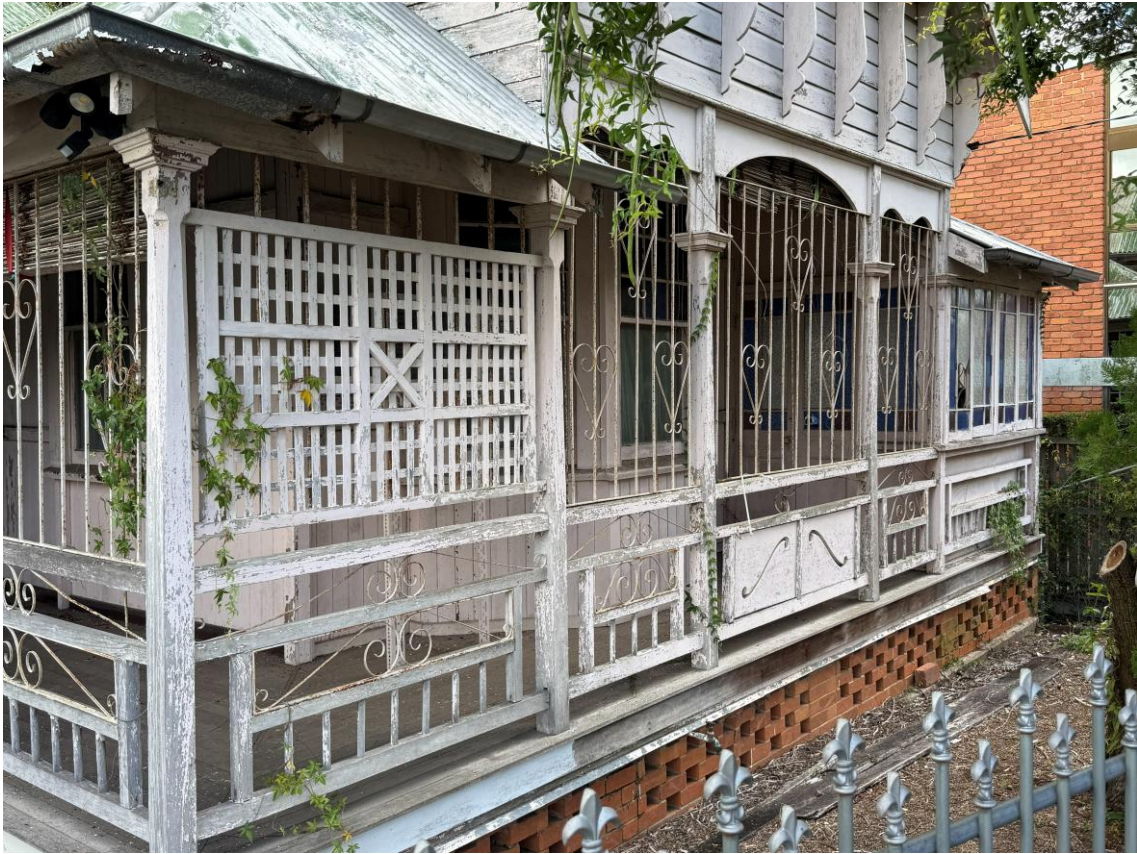
Figure 3: Perrot Street Frontage (3)
