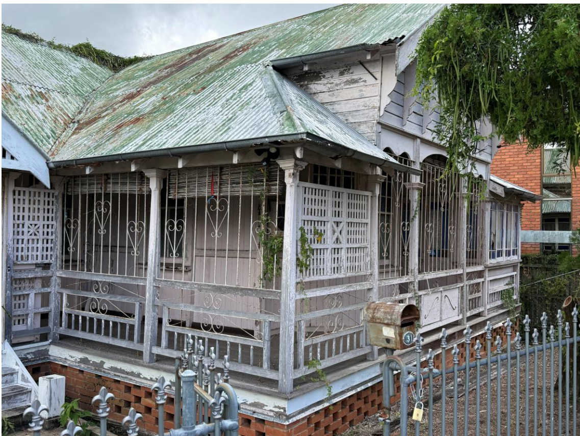
Figure 4: Perrot Street Frontage (4)
